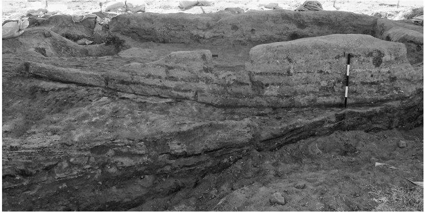
Figure 27.19. External face of west wall showing the building constructed on the uneven underlying midden deposits (Photograph by Freya Sadarangani).
