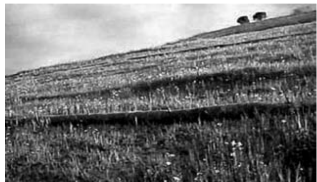
Fig 3.1 Stabilization - restoration of disordered soils using wood fences and for protection (Paylidis et. al, 2012).
