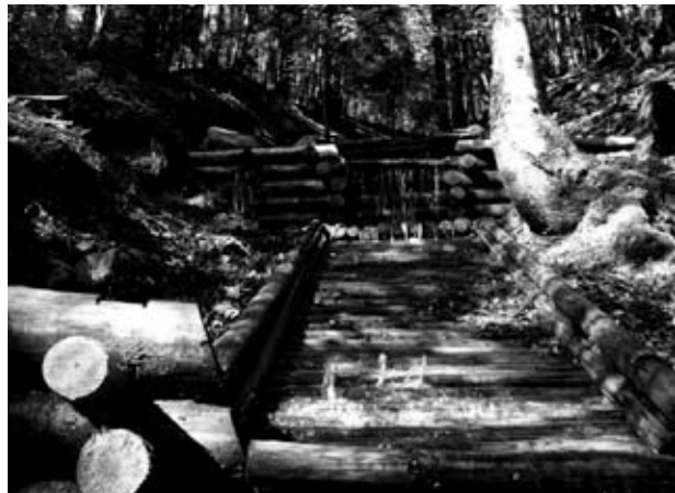
Fig. 3.4 River restoration work using belts, stones, wood, and plant material for slope and river bed protection (Pavlidis, 2012).
