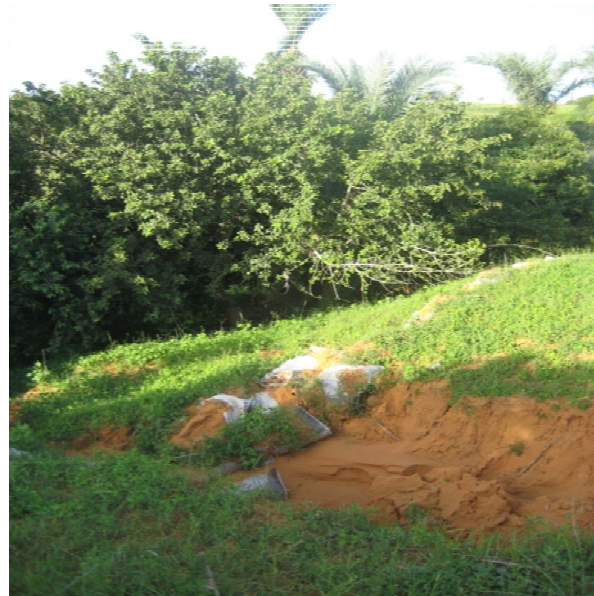
Figure 1. Anti erosion measure in Biidi-2
