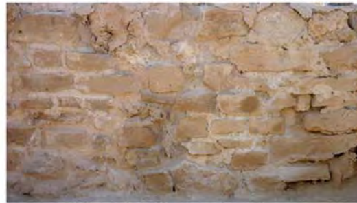
Figure 15: Test fields with NHL mortar at Eastern part of tower structure (Roman numerals refer to sample numbers in table 6)
