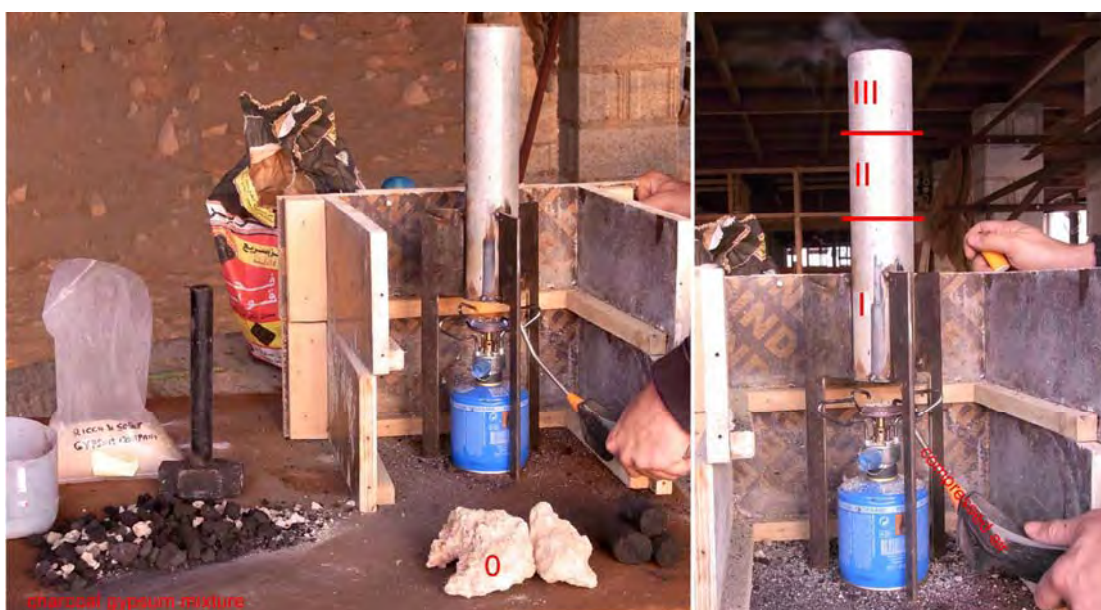
Figure 15: Tube-like experimental kiln for the burning of gypsum
