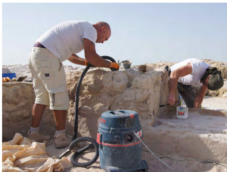
4. Remove loose materials and clean with an industrial hoover.
