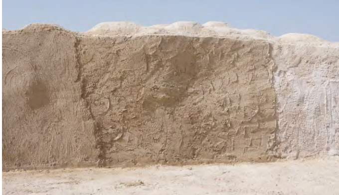
1. Building up of mortar layers
