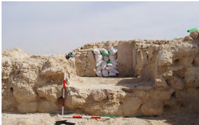
Window at palace before consolidation (01/2012)
