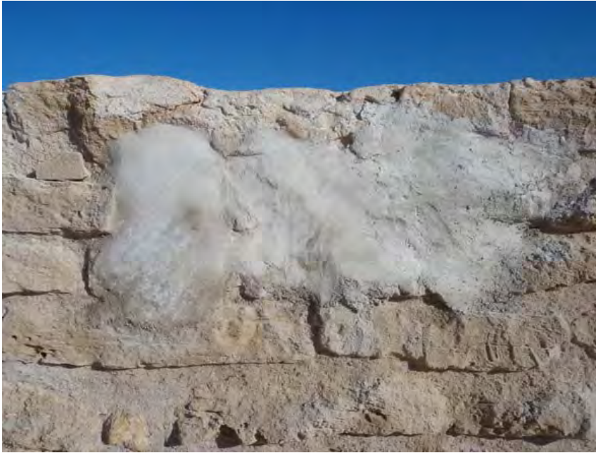
Figure 22: Gypsum plaster at test wall in the North Field
