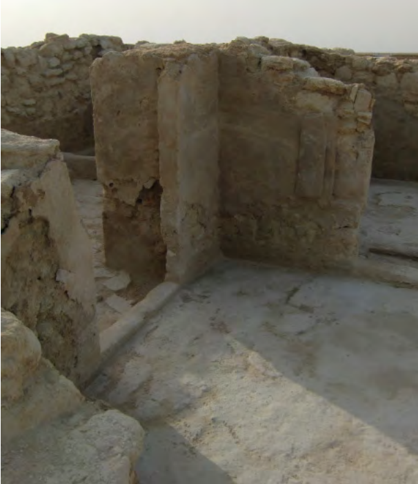
Historic (anhydrite) plaster floor at the palace; (03/2010).
