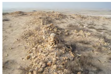
Al Jumail, compounds in the northern part of the village. Ruined walls made of stone and mud mortar
