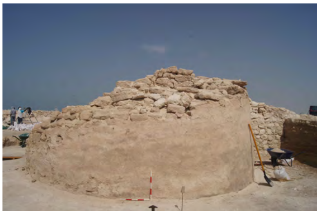
Tower (4012) at palace before consolidation (2011)
