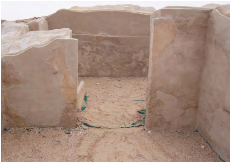
Comparable situation in the Palace (ZUEP04) after consolidation and re-plastering. Historic plaster remains were consolidated and integrated in the plaster surface.
