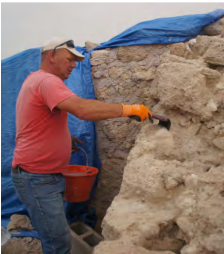
6. Pre-watering of wall stones before mortar is inserted.
