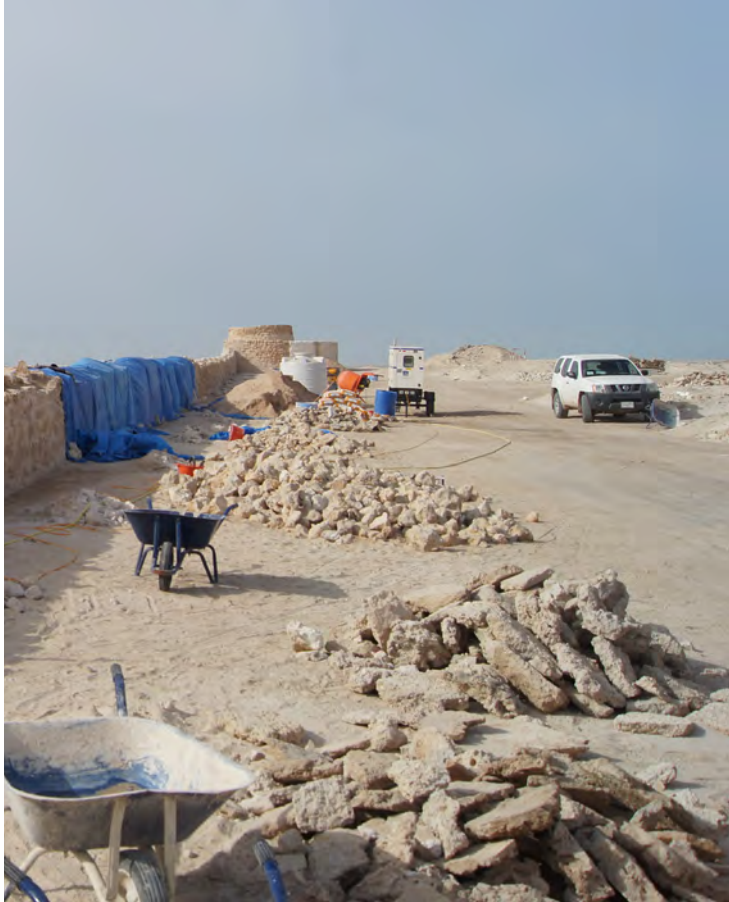
5. Pre-select stone material according to quality and (possibly) field of application
