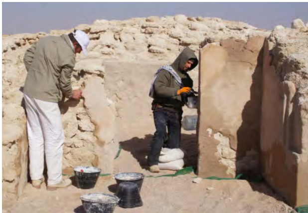
Consolidation of Plaster surfaces see Fiche No. 4.1
