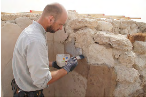
Consolidation of Plaster surfaces see Fiche No. 4.1
