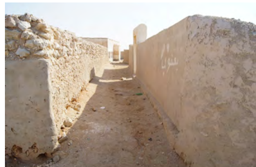
Al Jumail, courtyard walls in the village erected partly in 2009. Left: top of the wall made of stones with earth mortar, no plastering at all. Right: the fine, thin layer of mud plaster covering the rounded wall.
