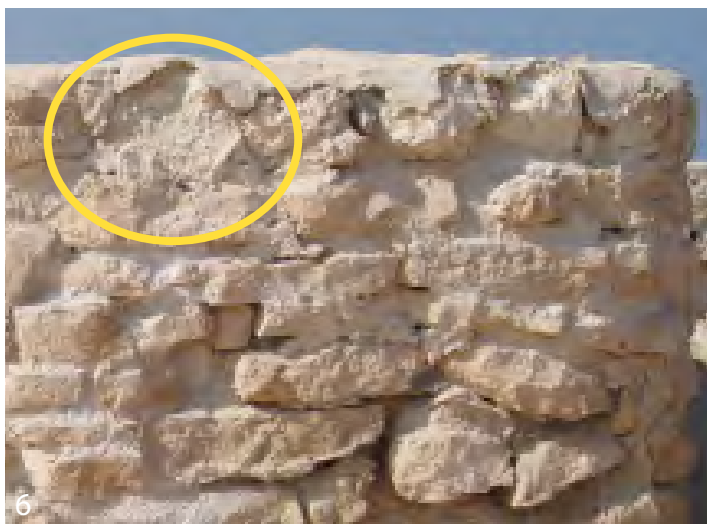
First mortar tests at Al Zubarah in November 2009: Soil mortar mix with the soil from the site. 1. Wall in QMA2 before test; 2. Close up on wall; 3. Mixing soil mortar; 4. Re-pointing of joints and fill of voids; 5. Fill hole to stone surface; 6. Same situation in December 2010.
