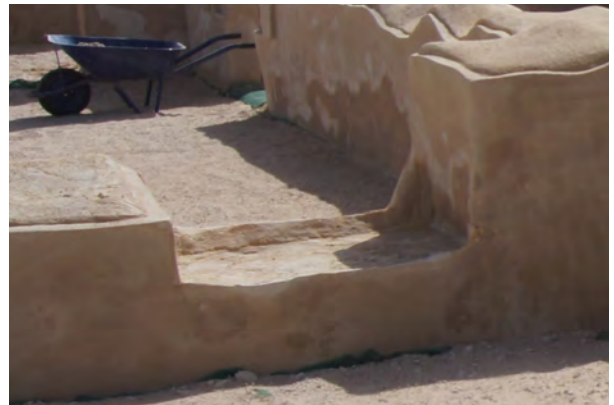
Window at palace after consolidation (03/2012)
