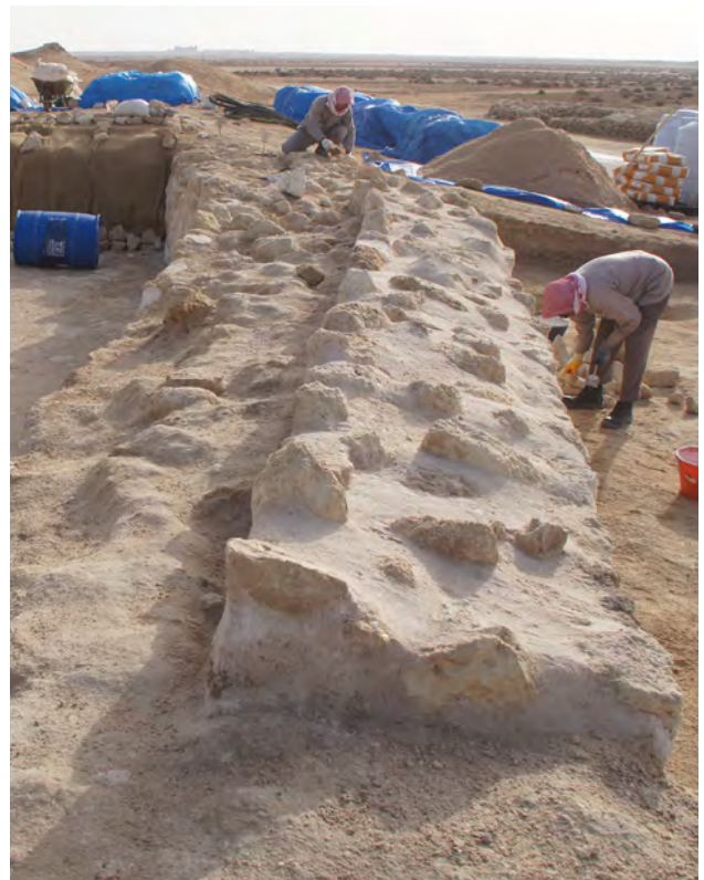
Town wall segment at tower 4012 (ZUEP04) in March 2012 (VAR. 2).
