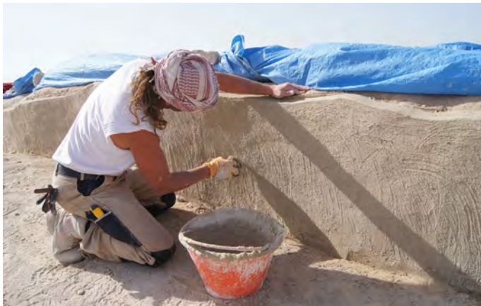
2. Applying final render by hand with gloves...
