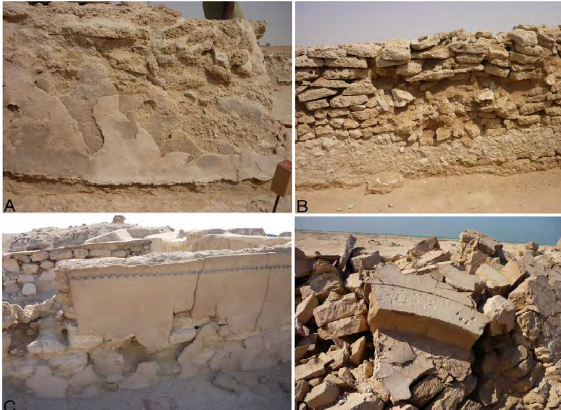
Figure 11: Sampling localities at Freha and at Al Zubarah. A. Double-layered wall plaster at Freha mosque, B. wall mortar at Freha mosque, wall plaster at Al Zubarah city, South field R.005, wall C (C) and Al Zubarah city area of consolidation (D)
