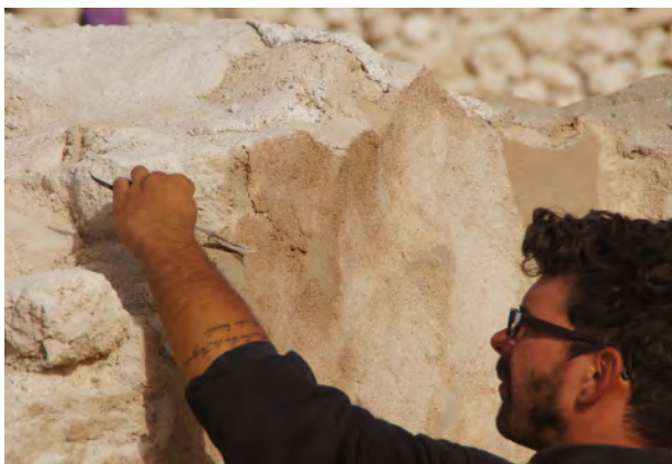
Cementing of Cracks see Fiche No. 4.3
