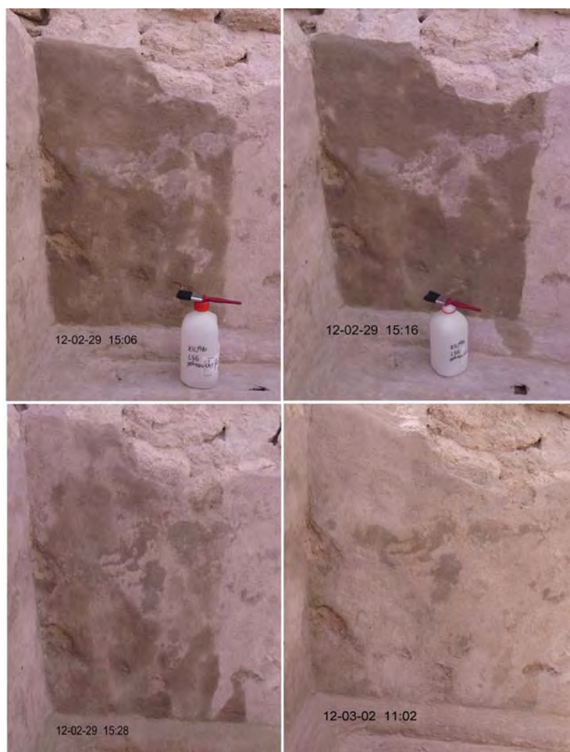
Figure 25: Consolidation test with Xilan® at wall plaster (gypsum) in room with mastaba at EP 04
