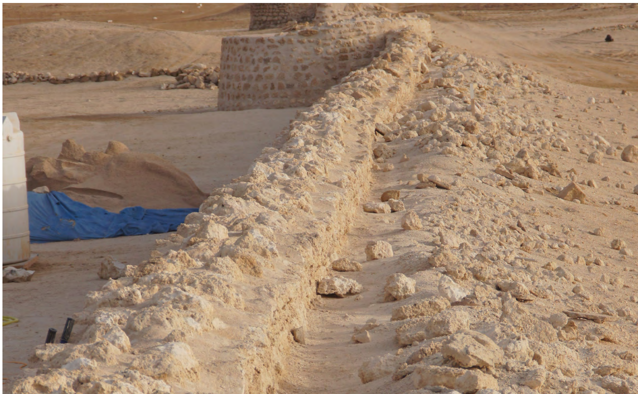
Town wall segment 8/9 with re-shaped crown in March 2012 (VAR. 1).
