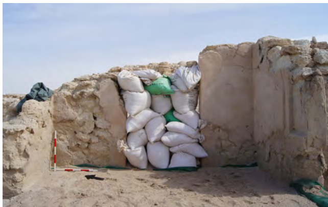
Doorway at palace before consolidation (01/2012)
