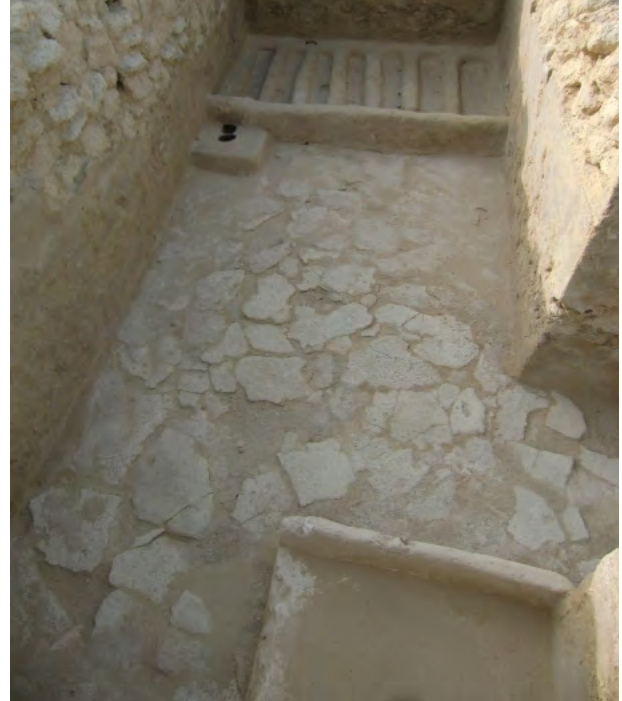
Pavement made of conglomerate stone slabs; This kind of pavement can also be found under the plaster floors as an underbed (03/2010).
