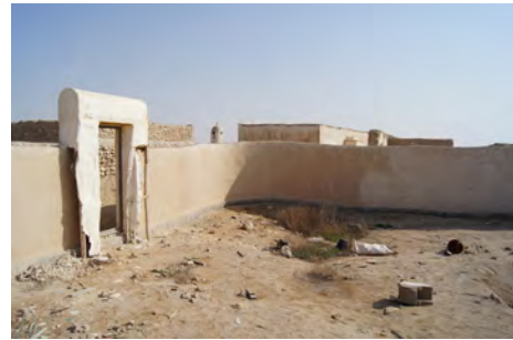
Al Jumail, S42, courtyard walls erected in 2009; the gate made of textile and gypsum plaster
