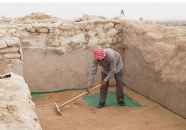
Cleaned floors should be covered by mesh or geotextile before a layer of fine sieved soil or better quartzsand is placed on. The layer of sand should be around 5 cm.
