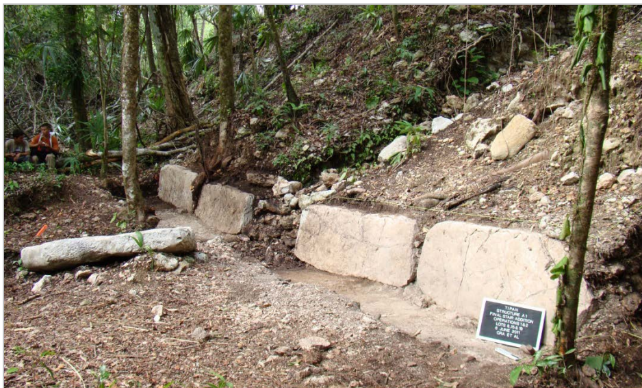
Figure 3. Photograph of the massive facing stones forming the west face of the platform constructed at the base of Str. A-1's Late Classic period outset axial stair at Tipan (photograph by Christopher R. Andres).
