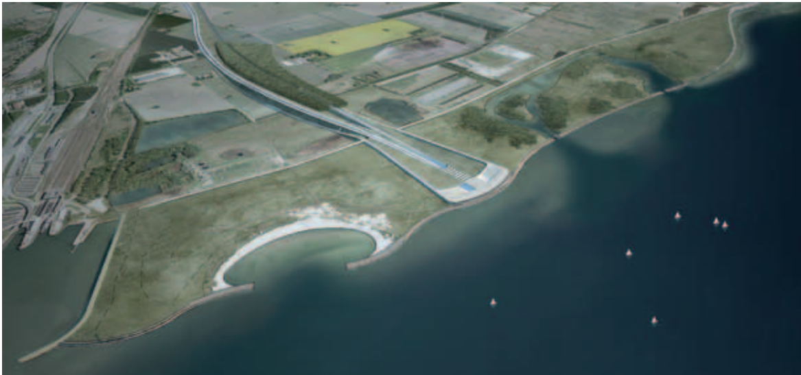
Figure 9. The tunnel entrance on the Danish side of Fehmarnbelt includes a control and monitoring centre in the portal building.
