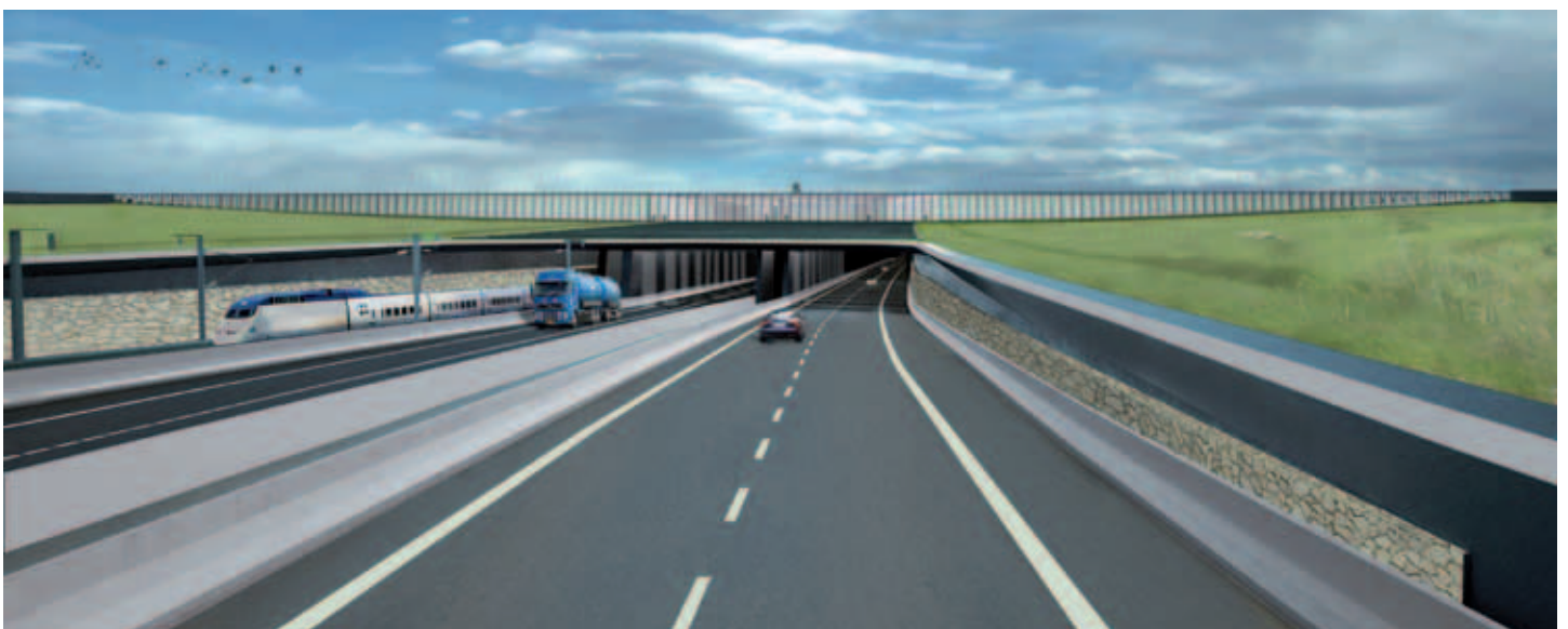
Figure 4. The approach ramp and portal structure on the Danish side of a Fehmarnbelt tunnel with the control and monitoring facilities seen from the north towards the south.
