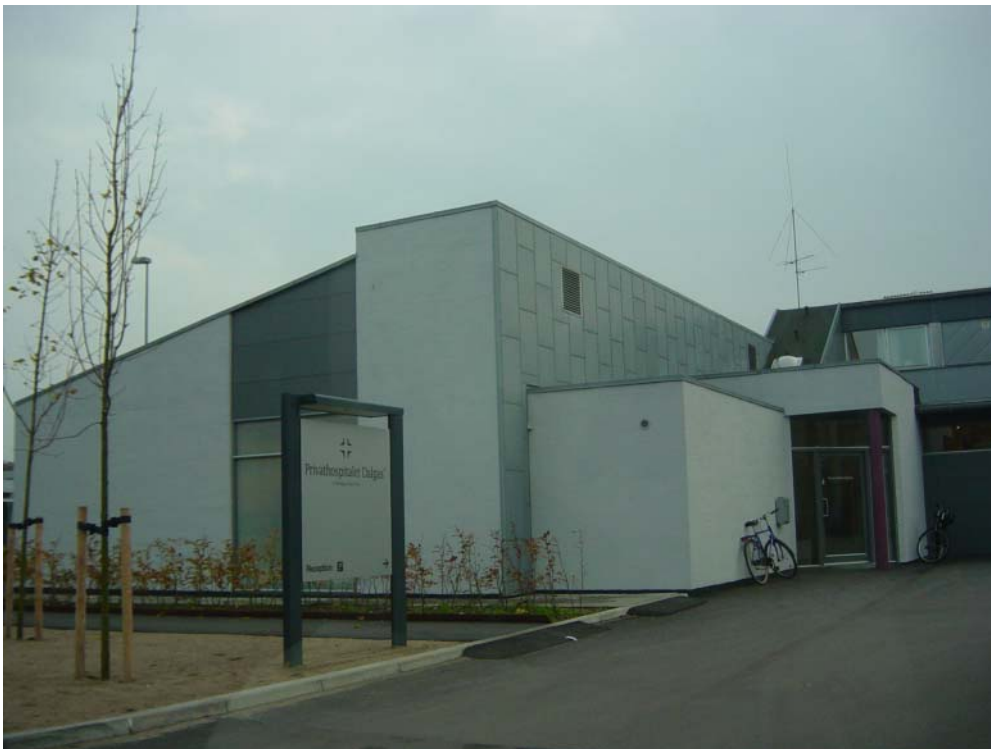
Figure 34. From textile to hospital Buildings from the former ELAS rubber products firm are remodelled into the Dalgas private hospital.
