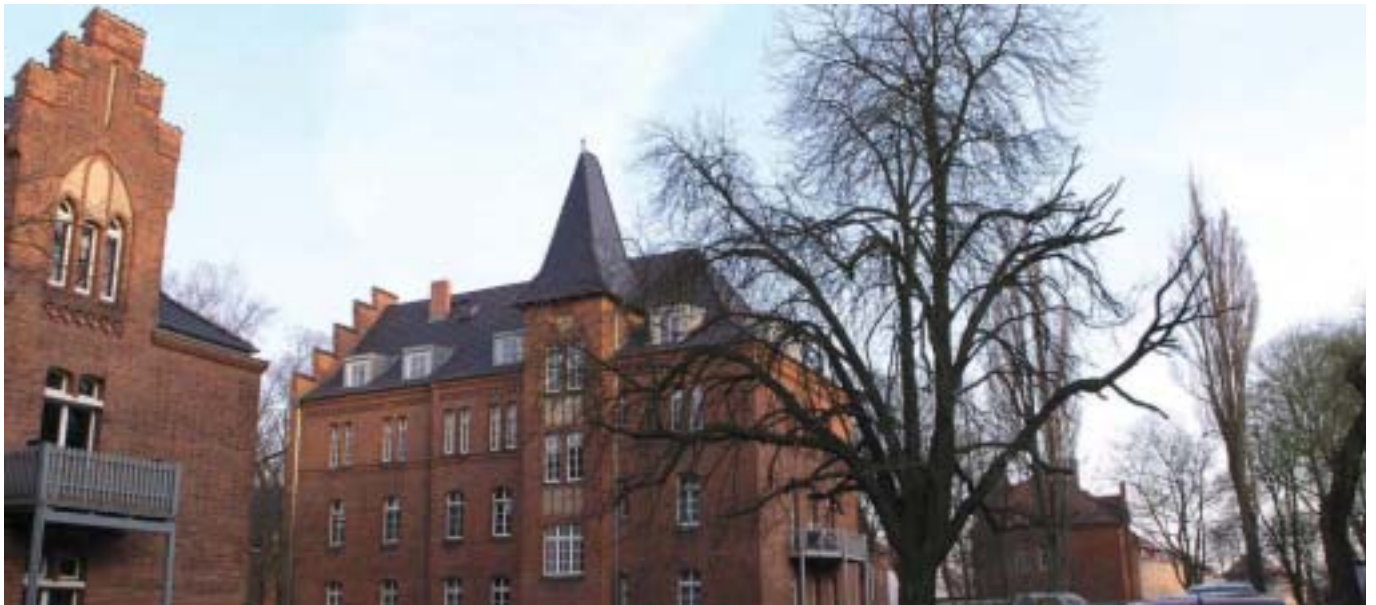
Jüterbog II. From military barracks to housing units.
