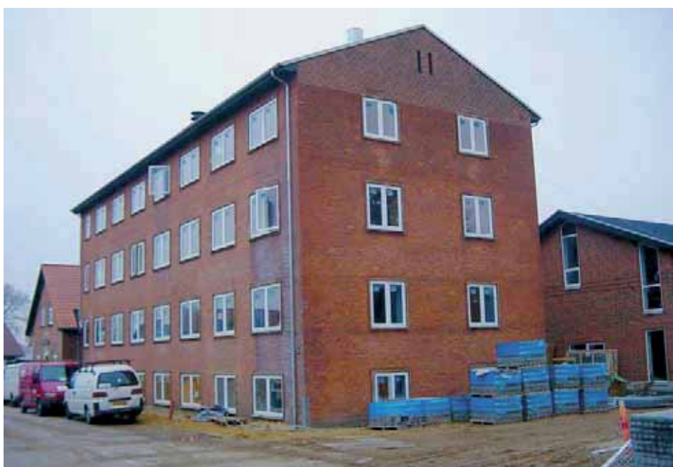
Figure 1. From textile to dwellings. The former garment factory, Hammer Thor is remodelled into apartment units.
