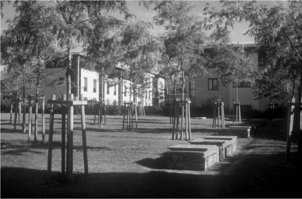
Fig. 20 Edward Square, social housing initiated through the projects.
