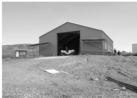
Fig. 1.3. The boat house in Daneborg is situated just at the shore-line. The windows in the left side of the picture is leading to a combined laboratory and office facility with electrical heating. Photo Morten Rasch.
