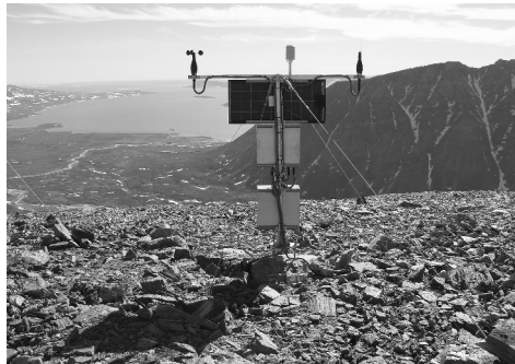
Fig. 2.3. The new meteorological station (M6) on Domebjerget is located 1282 m a.s.l. Snow depth is measured from a separate mast whereas all other parameters are measured from the main mast where also the solar panel and two enclosures for datalogger and batteries are mounted.
