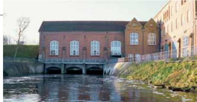
Following the construction of the Tangeværk hydroelectric power station in the upper reach of the River Gudenå between 1918 and 1920, salmon were unable to reach their spawning grounds. Only a few years later, salmon were extinct in this river.
