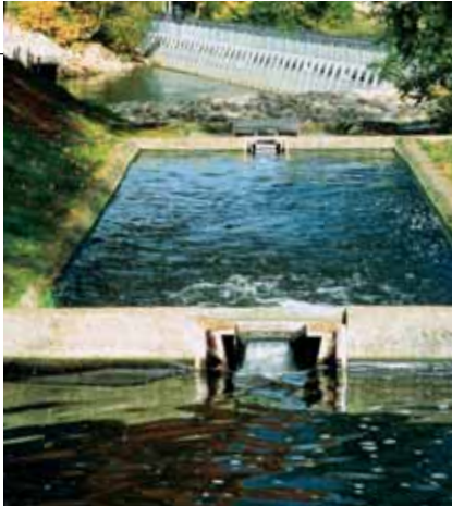
A fish guidance fence and fish ladder at the Tange Hydropower Dam on the River Gudenå.
