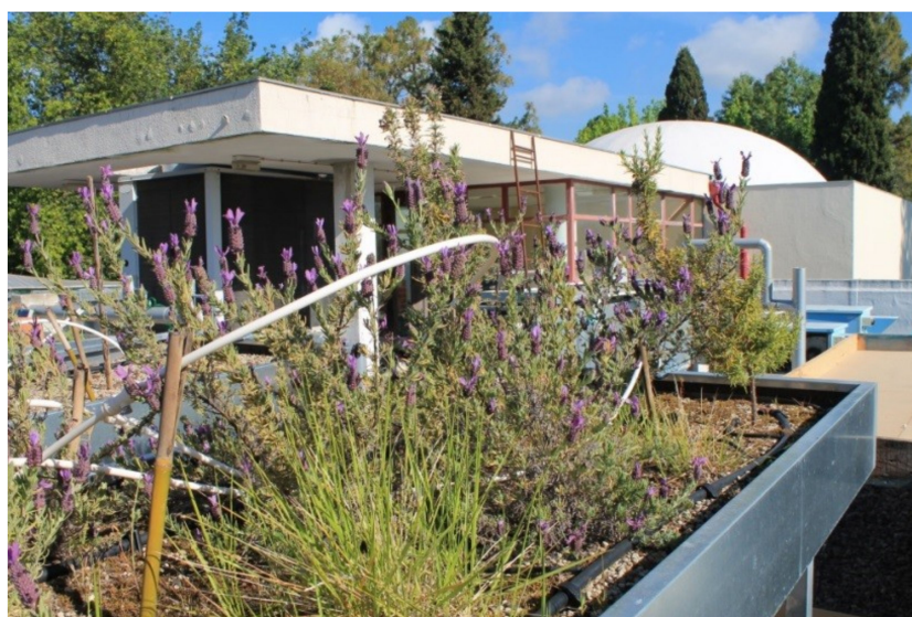
Figure 3. Test bed with vascular plants and mosses at the rooftop of the Herbarium building at Instituto Superior de Agronomia, University of Lisbon, Portugal.
