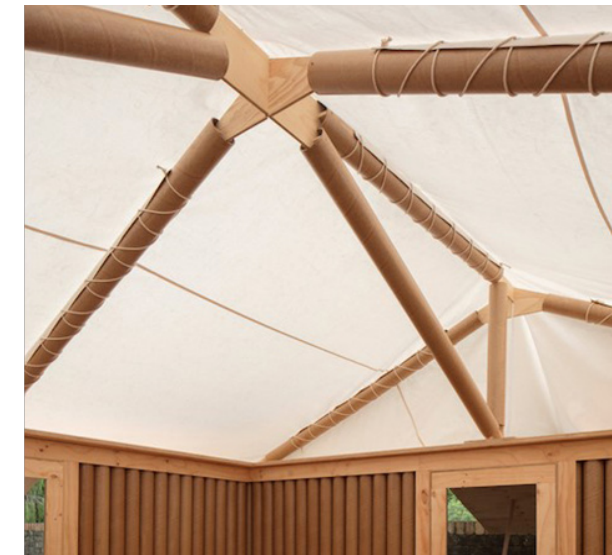
Paper log house, Shigeru Ban, Brett Boardman
