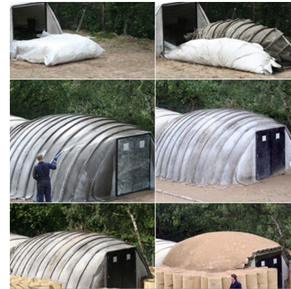
Concrete canvas shelter, Will Crawford y Peter Brewin
