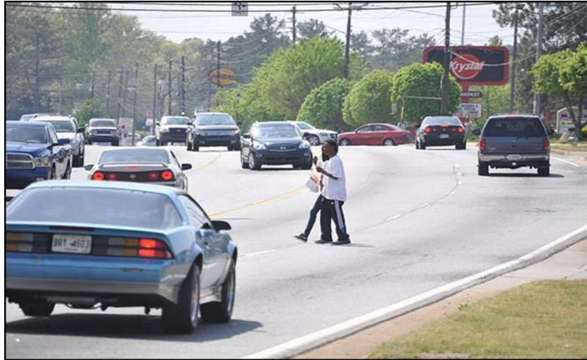
Figure 6.25: Pedestrians crossing a road with a painted two-way left-turn lane median (S. L. Davis, 2014).
