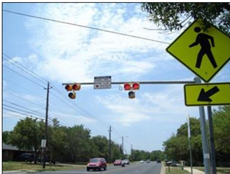
Figure 6.20: Example of a HAWK beacon in conjunction with a pedestrian crossing warning sign (Fitzpatrick et al., 2016).
