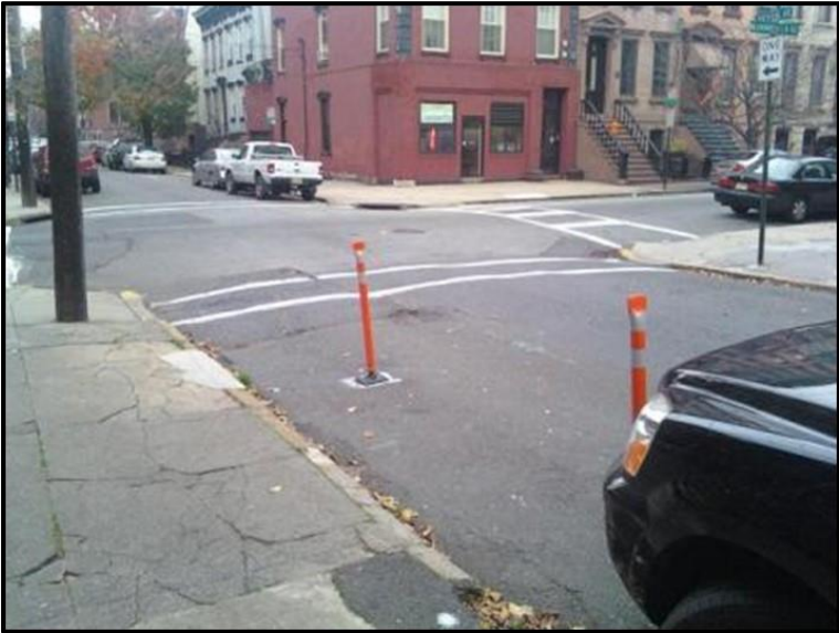
Figure 6.17: Daylit intersection through the use of vertical delineators (Sacs, 2009).
