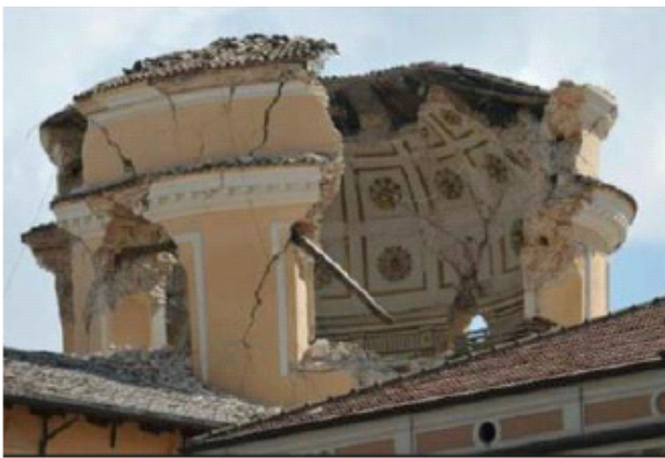
Fig. (2). Dome and drum of the Anime Sante Church in L'Aquila after the earthquake of 2009.
