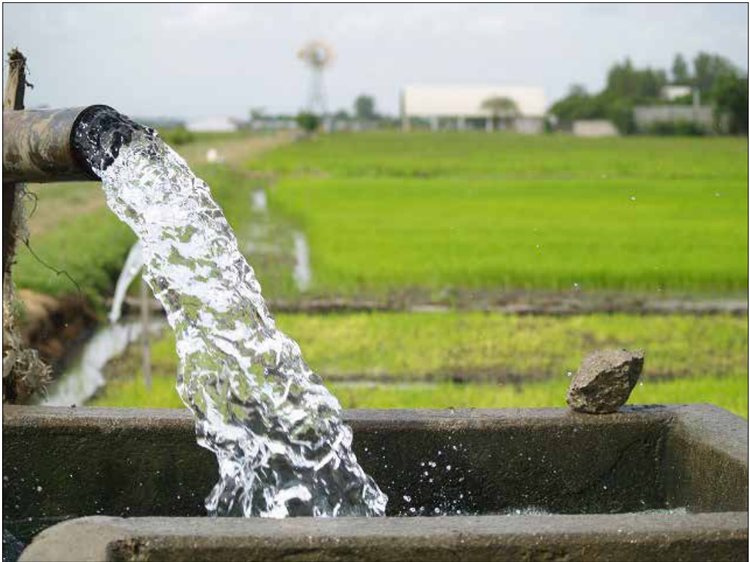
Figure 2.25. AWD using pump irrigation in rainfed lowland helps in reducing water consumption without affecting crop yield
