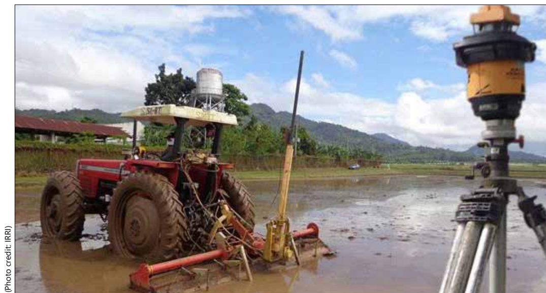
Figure 2.16. A laser-controlled land leveling set-up in the field
