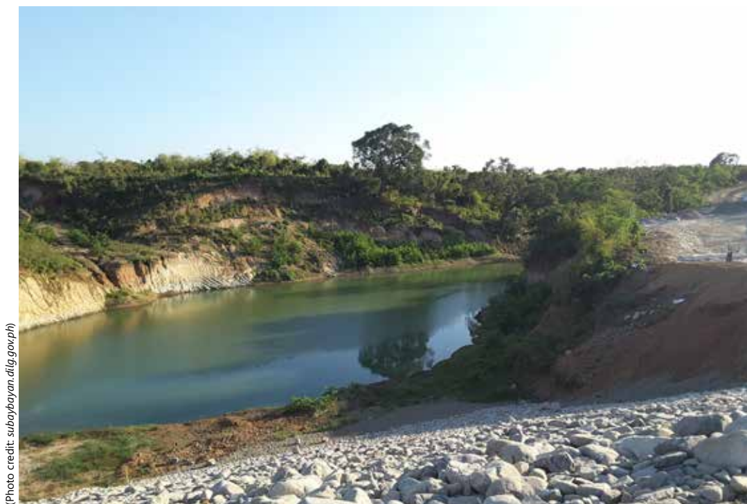
Figure 2.27. Water harvesting in micro-watershed is done by constructing earth embankments called small water-impounding structures
