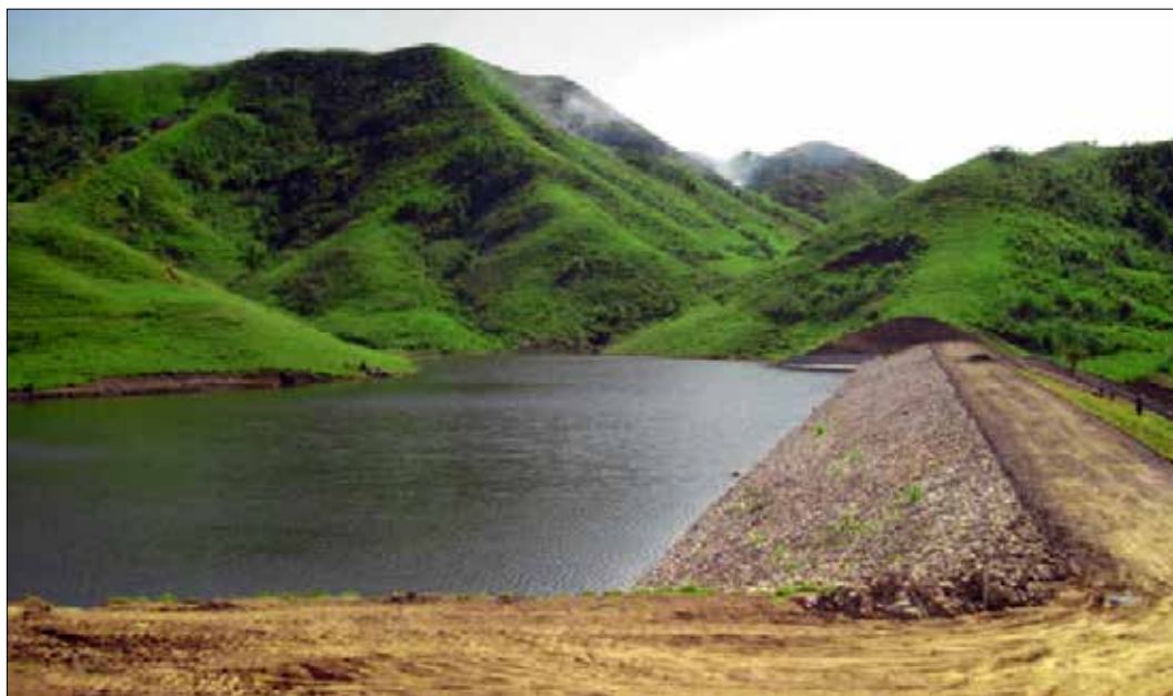
Figure 1.7. A watershed with water impounding structure as source of irrigation for the lowland areas
