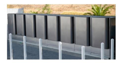
Picture 5.35 Bloom Energy ES5 – YA8AAN 300 kW, each producing power at 300 kW [Bloom Energy, 2019]
