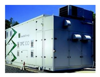
Picture 5.36 FuelCell Energy DFC 300 MCFC power plant [FuelCell Energy, 2018]
