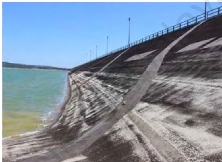
Figure 2.1: View of Lentini earth-fill dam (Castelli et al. (2016))
