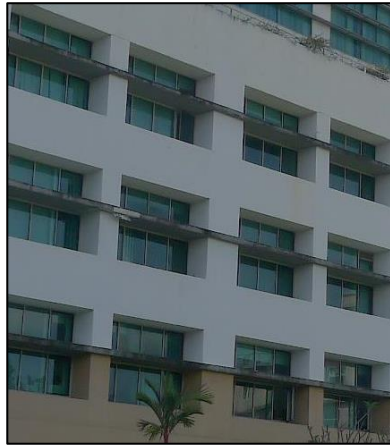
Figure 4.19: Punch-hole windows on the North façade
