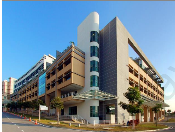
Figure 4.14: Exterior view of LEO building (Source: www.greenbuildingindex.org )
