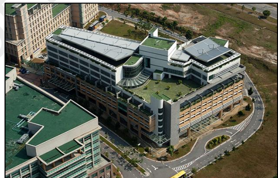
Figure 4.17: Aerial and façades view of LEO building (Source: http://www.p-perdana.com/ )
