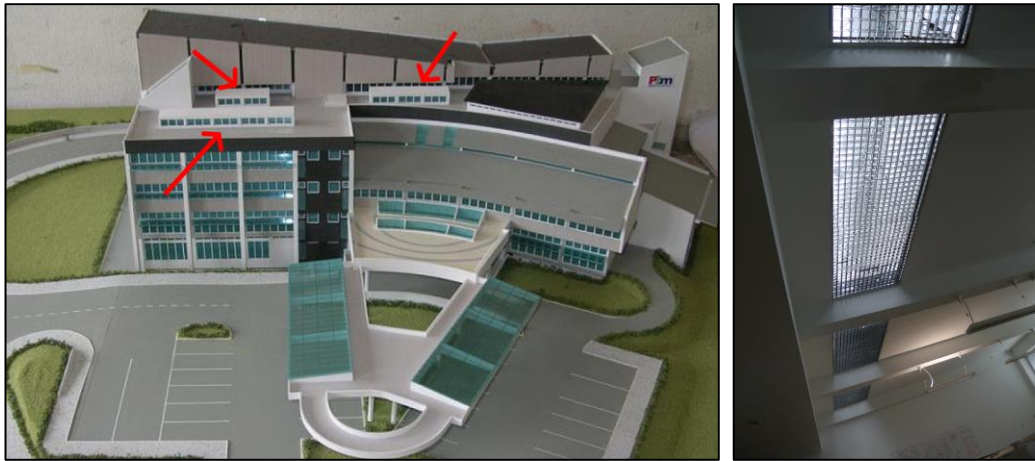
Figure 4.31: The location of roof light trough system on the flat roof and the interior light diffuser
