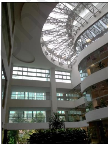
Figure 4.21: View of the middle atrium in LEO building
