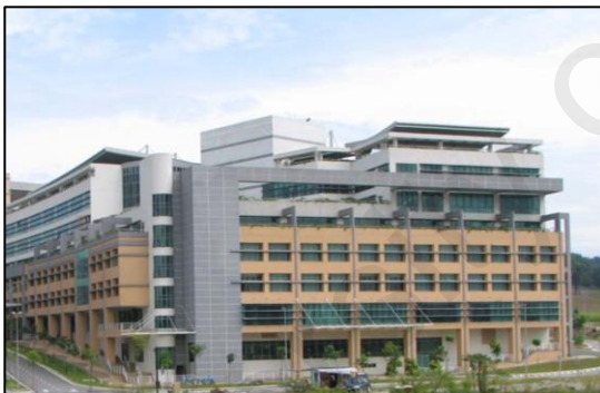
Figure 4.16: East façade view of LEO building (Source: Roy et al., 2005)
