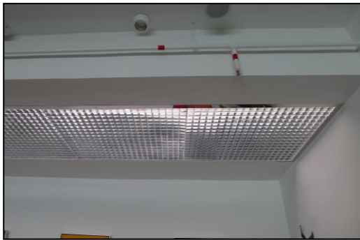
Figure 4.8: View of roof light-trough from the interior space
