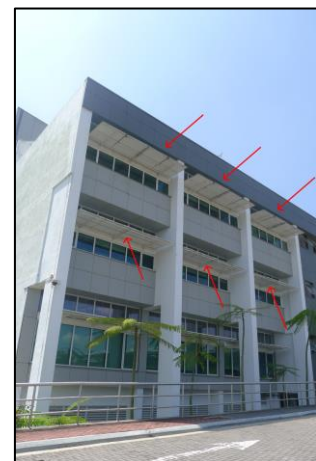
Figure 4.30: Location of the mirror light shelves on GEO building's North façade
