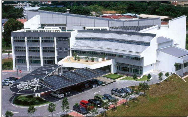
Figure 4.24: Exterior view of GEO building (Source: www.greenbuildingindex.org )
