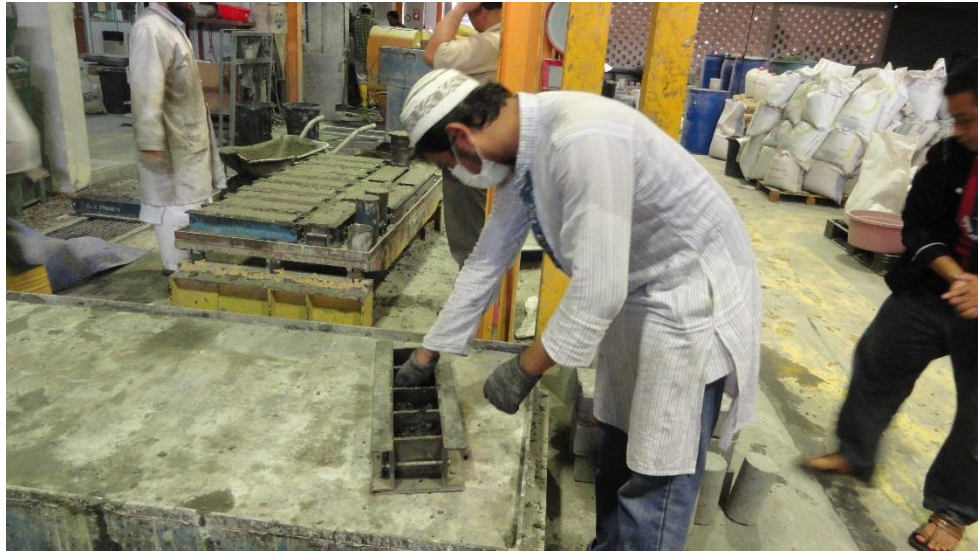
Photo B.13: Preparation of moulds for casting
