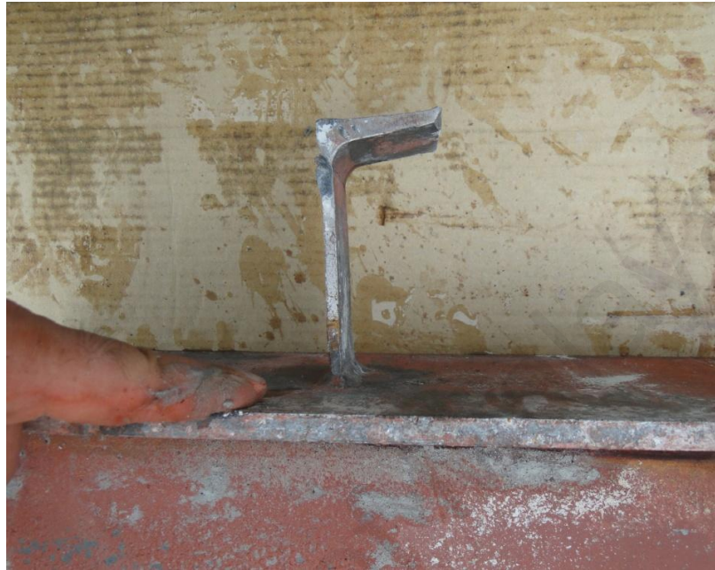
Figure 2.7: Typical angle shear connector
