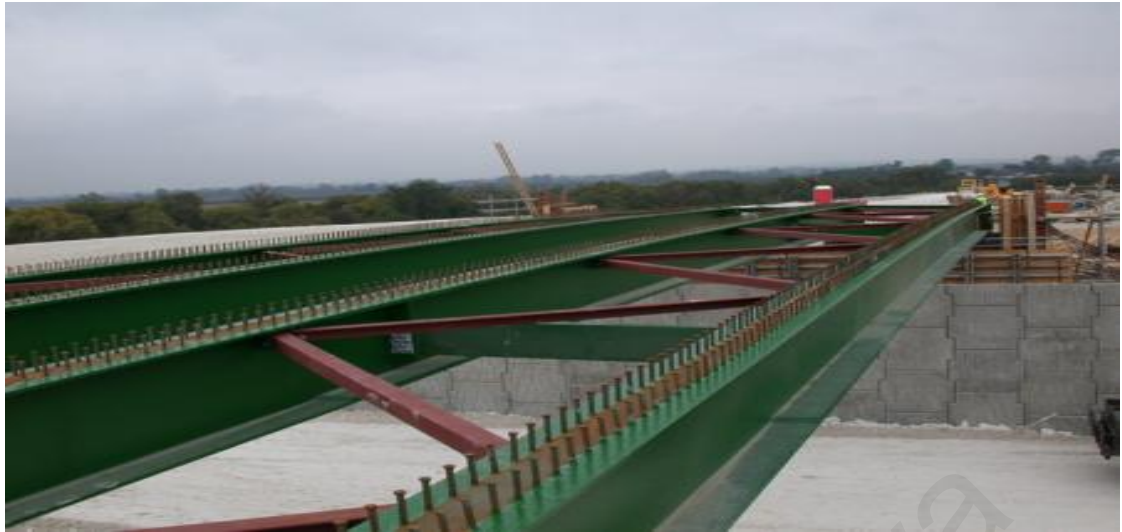
Figure 2.3: Headed stud shear connector
