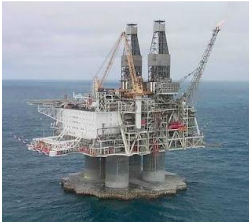
Figure 2.2: Concrete gravity structure (MOG, 2010)
