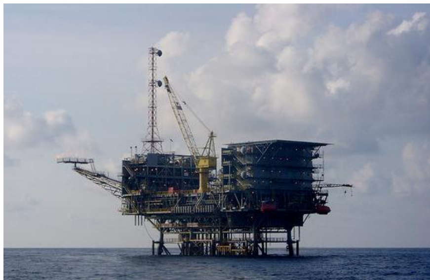
Figure 2.1: Fixed offshore platform (MOG, 2010)
