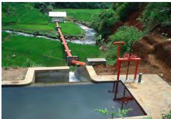
Figure 2.7: Run-of-River hydropower plant (Energylopedia, 2016)
