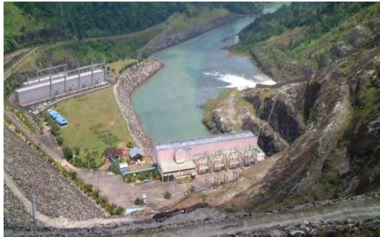
Figure 2.5: Kenyir (Sultan Mahmud) Hydroelectric Power Project Malaysia (KualaLumpur-Post, 2016)
