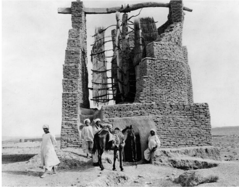
Figure 2.2 Sistan turbine for milling grain in Afghanistan (Hau, 2006).
