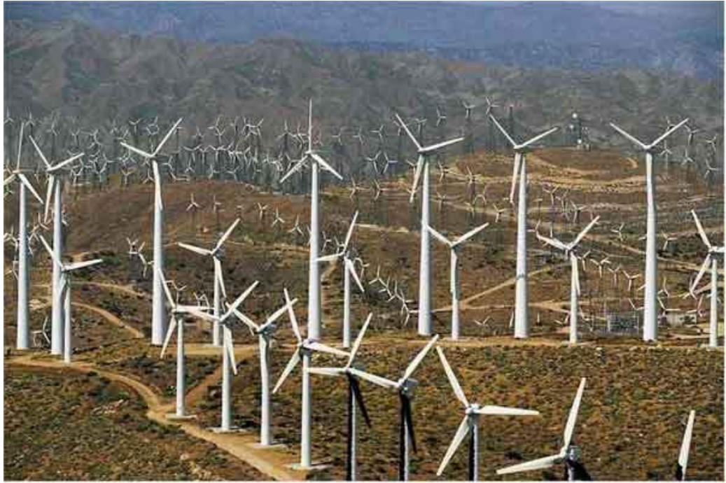
Figure 2.1 Wind farm for electricity generation to large utility grid. The picture shows one of the largest on-shore wind farms is the Roscoe Wind farm in Texas, USA. The farm covers an area of 155 square miles, and its 627 turbines have a total installed capacity of 780 MW (Roos, 2011).
