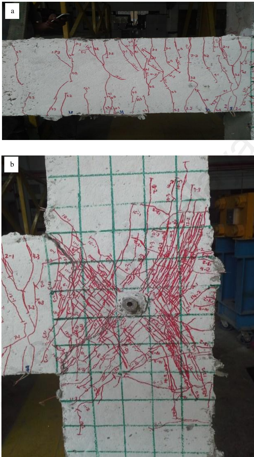
Figure 4.39 Crack propagation in (a) beam (b) joint region of PE 4 beam–column specimen
