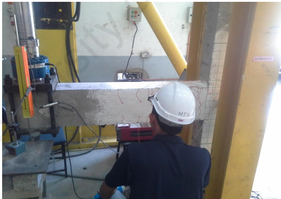
Figure 3.16: Observation of cracks propagation within the testing process
