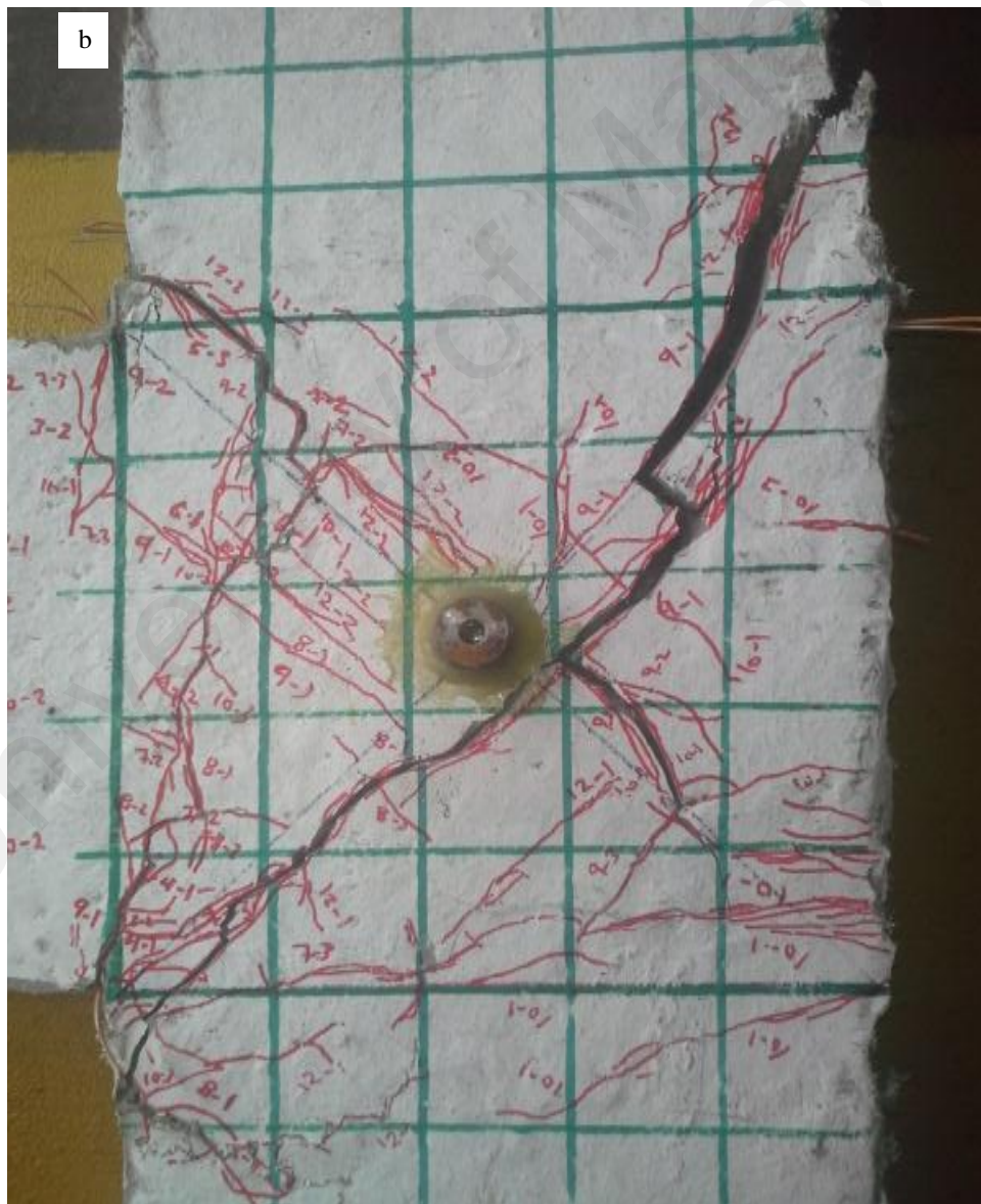
Figure 4.35: Crack propagation in (a) beam (b) joint zone of PVA 6 beam–column specimen
