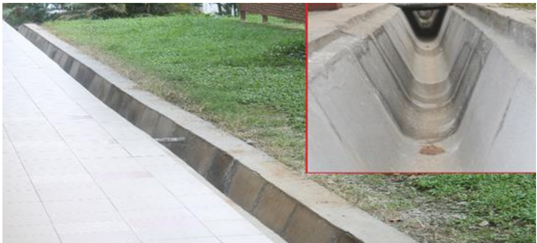
Figure 4-5: Example for Good Drains Restaurants; the images from outside and inside of the drain
