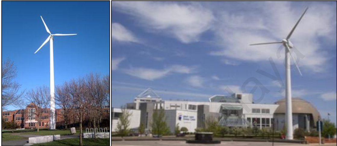
Figure 2.11 Stand-alone wind turbine at McGlynn Elementary School, Boston (left) and Great Lakes Science Center, Cleveland.
