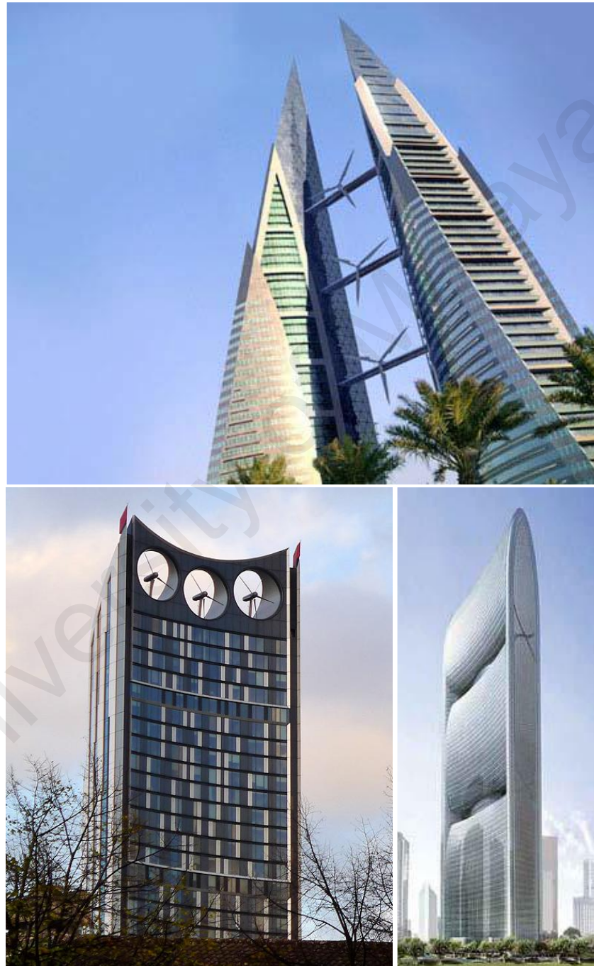
Figure 2.13 Top: Bahrain World Trade Centre ("Bahrain world trade centre (BWTC)," 2015); Bottom left: Strata Tower ; Bottom right: Pearl River Tower ("Pearl River Tower,").
