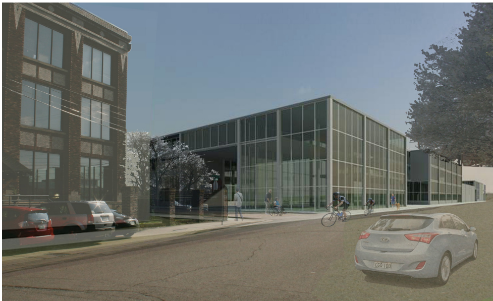
Figure 21: View towards lobby from North (page 18)
