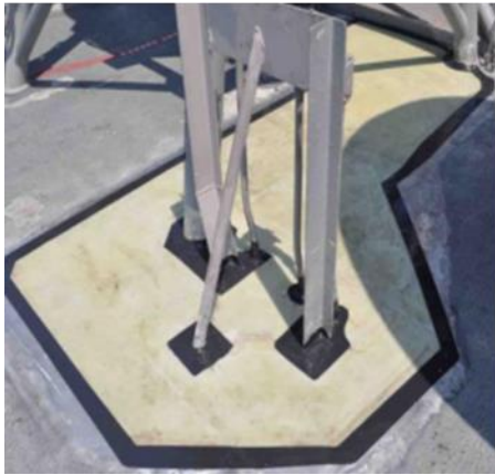
Figure 1. 2 Composite patches installed on marine aluminum structures [3, 4].
