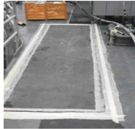
Figure 1. 2 Composite patches installed on marine aluminum structures [3, 4].
