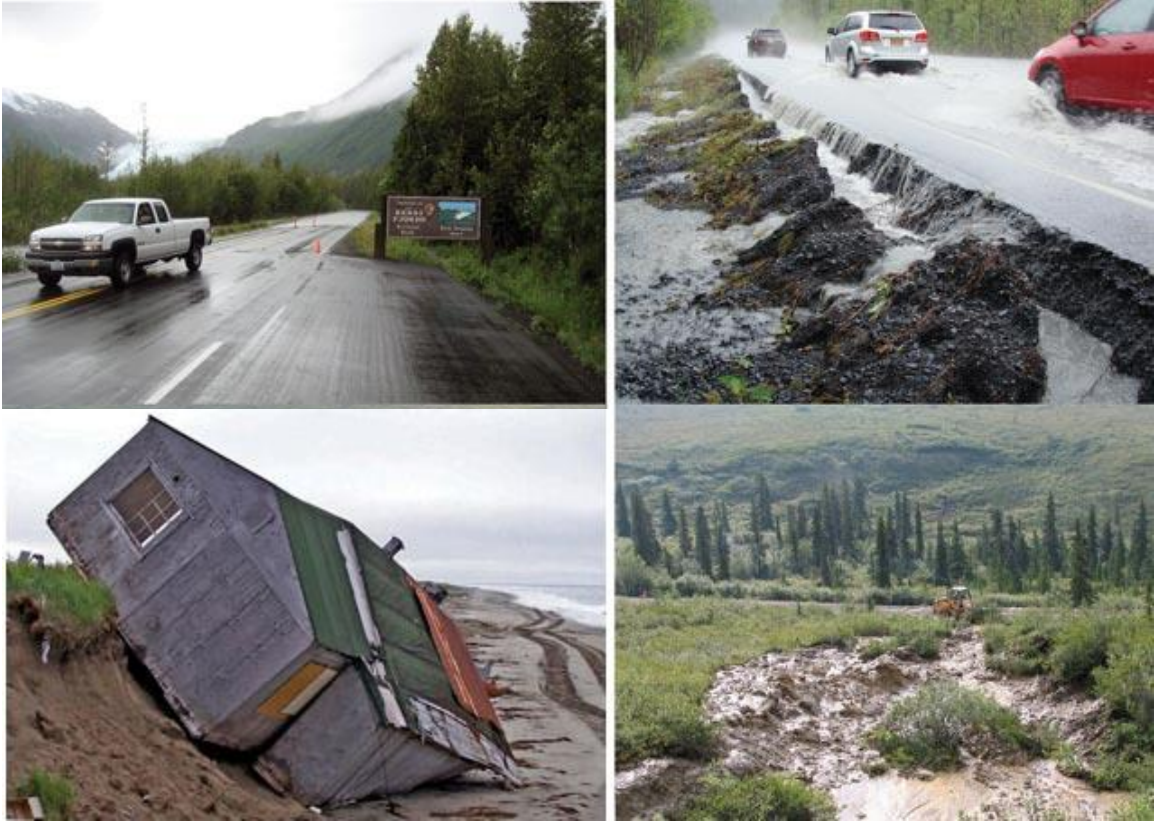
Figure 51: Images showing infrastructure damage due to thawing permafrost and eroding coastlines in the Alaskan Arctic
