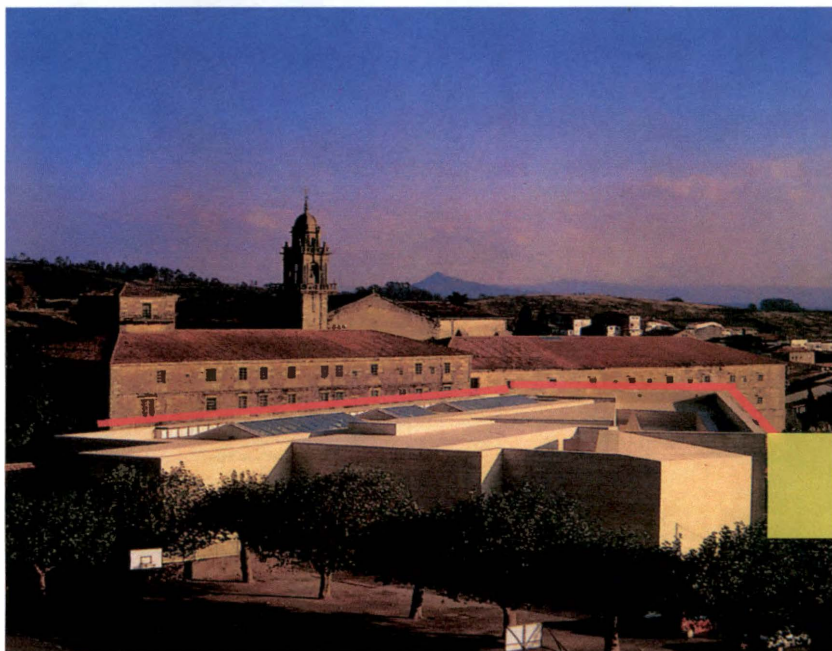
Figure 47 (A &B). The Centro Gallego de Art Contemporaneo, Santiago de Compostela, Spain by Alvaro Siza. The line of tension between the abbey and the museum and the entry transition point of the museum.
