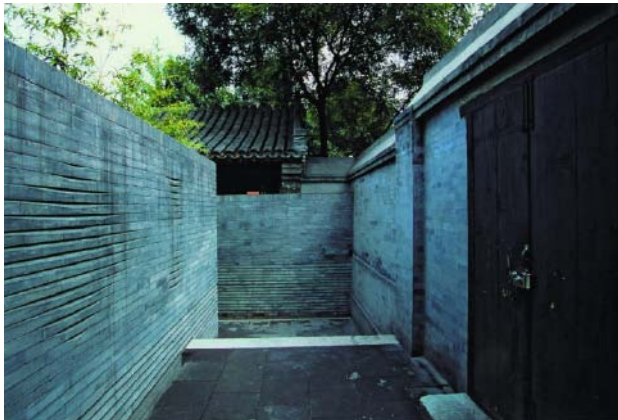
Figure 3-11: Screen Wall Source: ddyuanlin.com
