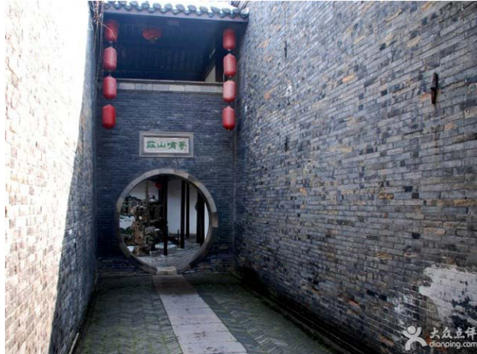
Figure 2-6: Wall for Private Mansion Source: s.dianping.com
