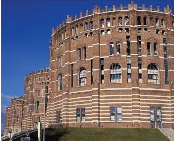
FIGURE 18. Gasometers after renovation (n.d.). [digital image]. Retrieved June 3, 2014 from http://21region.org/uploads/posts/2010-09/1284471179_3.jpg
