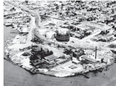
FIGURE 8. Decommissioned gas works plant
