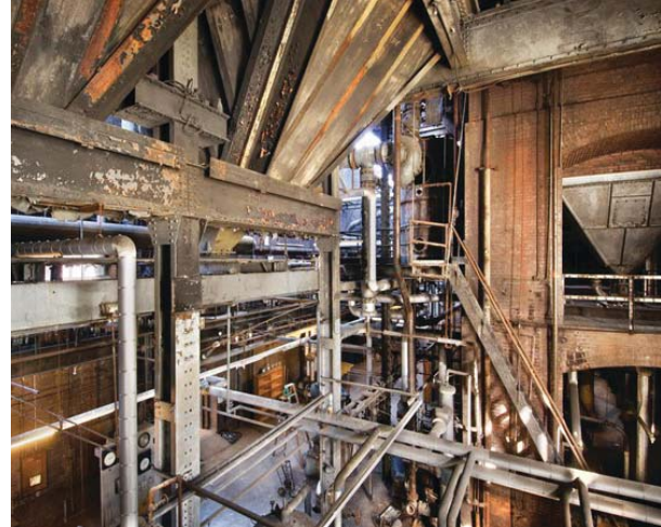
FIGURE 7. Architectural idea of Post-Industrial Harris, D.L. (Photographer). (n.d.). [digital image]. Retrieved June 20, 2014 from www.dbhms.com/about/articles/2010/CHshaw.html
