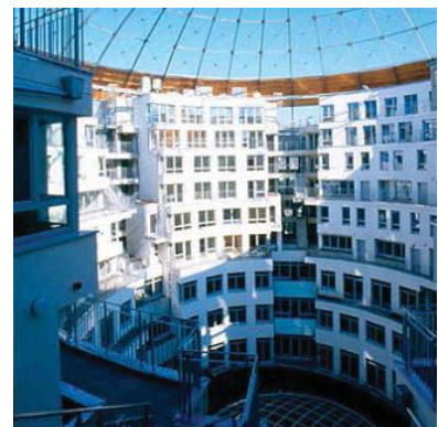
FIGURE 17. View into Gasometer C
