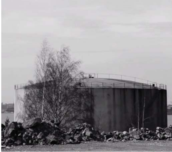
FIGURE 20. Silo 468 before renovation (n.d.). [Video Still]. Retrieved May 20, 2014 from www.idcol.com/286/silo-468
