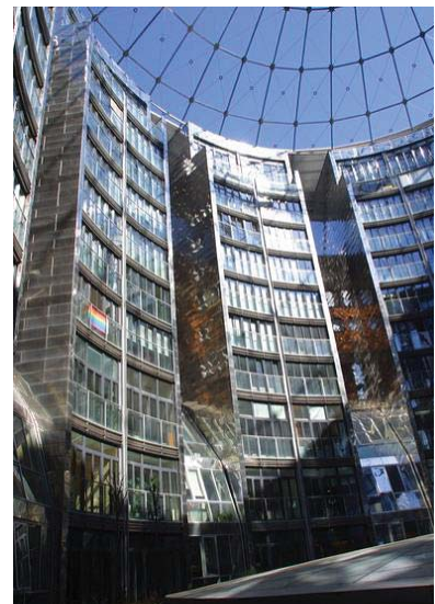
FIGURE 16. Inside Jean Nouvel's Gasometer A
