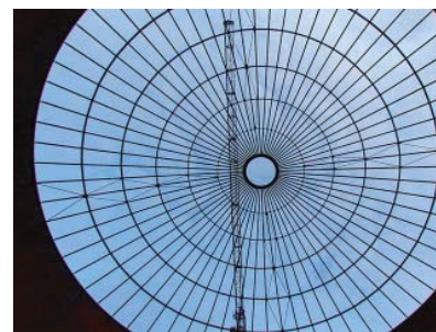
FIGURE 3. View through open silo roof structure to the sky
