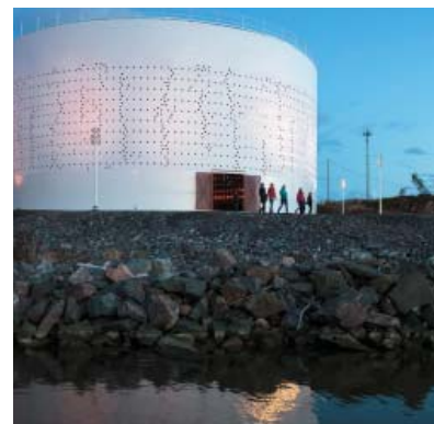
FIGURE 24. Exterior of Silo 468 (n.d.). [digital image]. Retrieved May 20, 2014 from http://www.designboom.com/architecture/lighting-design-collective-convert-silo-468-into-public-light-show-11-01-2013/
