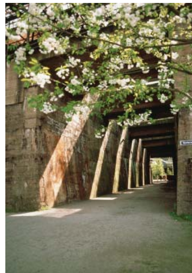
FIGURE 12. Blast furnace turned gateway entrance
