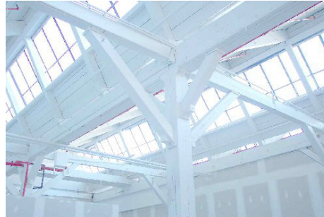
29. Plant Zero Arts Center Skylights Image Source: freenet.vcu.edu/arts/artspace/aboutus.htm
