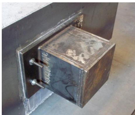
Figure 9. Impactor attached to the imbed plate.
