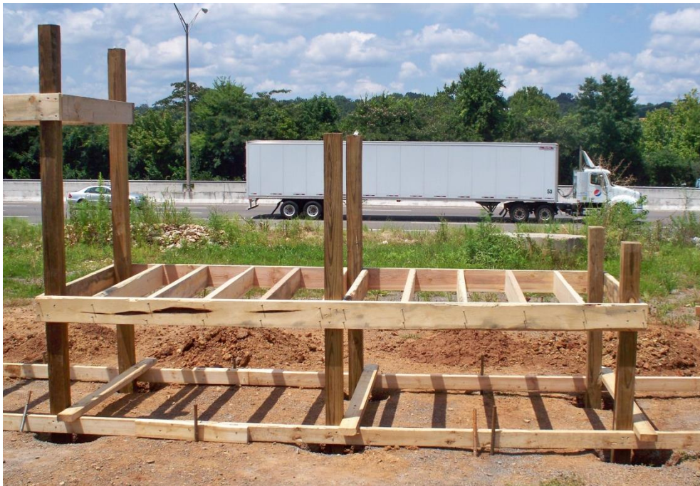
Figure 11. Lower work platform without decking and before casting of concrete.
