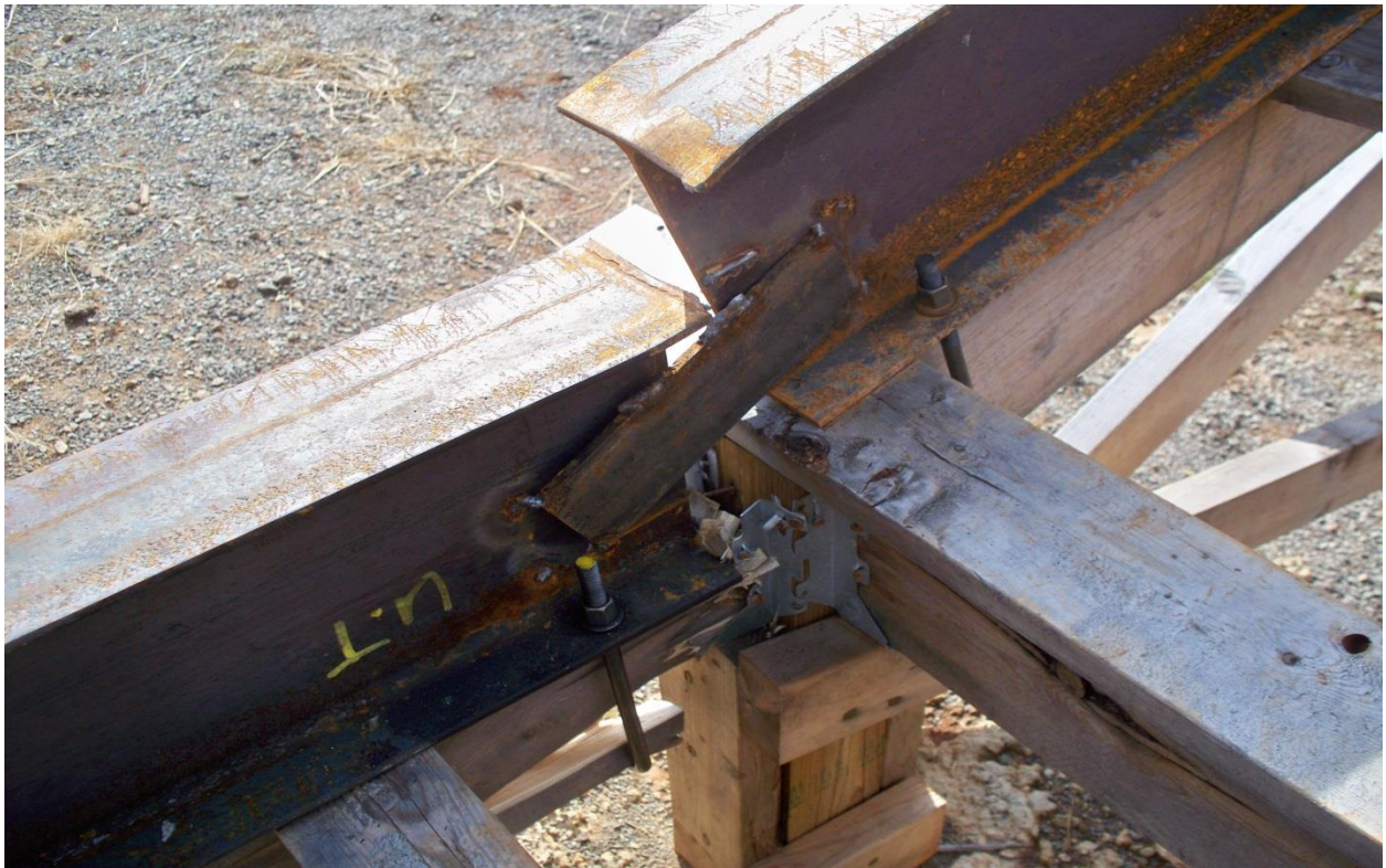
Figure 34. Damage to rails after testing.
