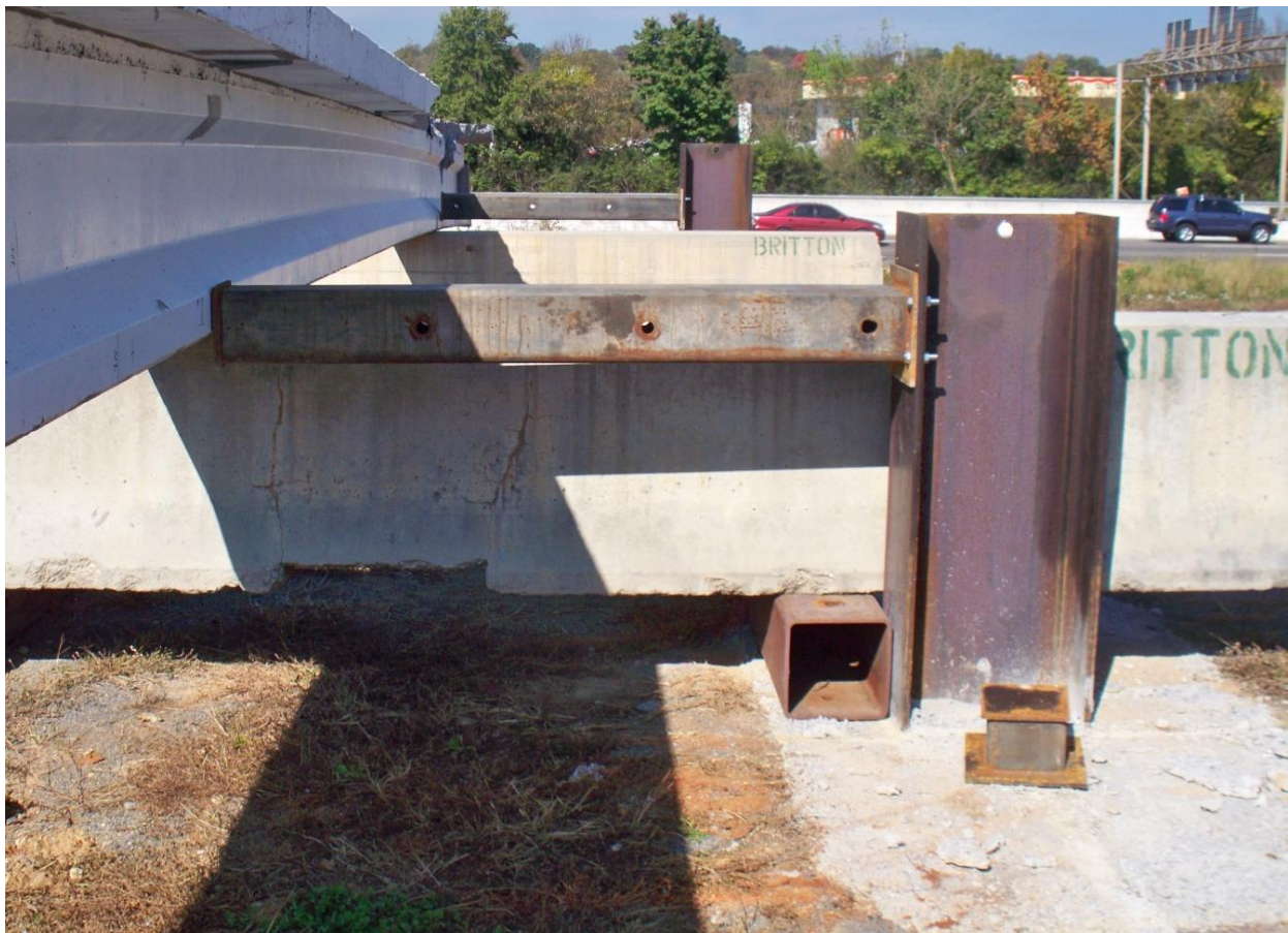
Figure 20. Completed backstop with footing beam and tube.
