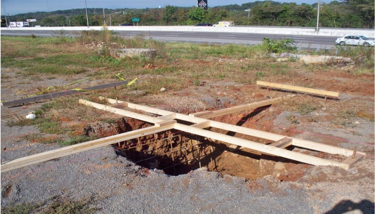
Figure 22. Guide system for steel beams.
