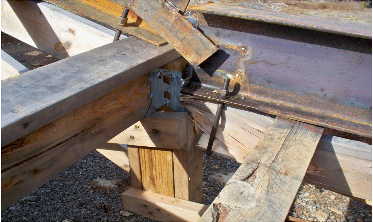
Figure 33. Damage to joists after testing.
