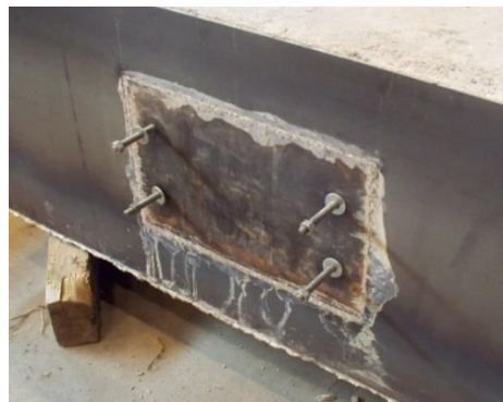
Figure 8. Imbed plate and attachment bolts.
