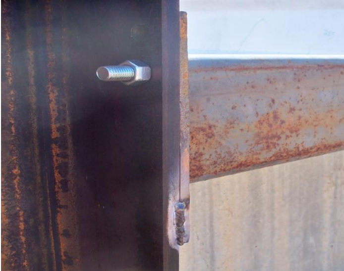
Figure 28. Connection of HSS tubes to vertical beams.
