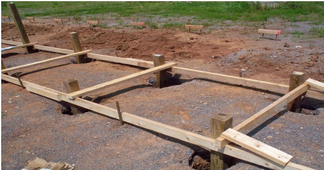
Figure 10. Posts screwed into guide boards.
