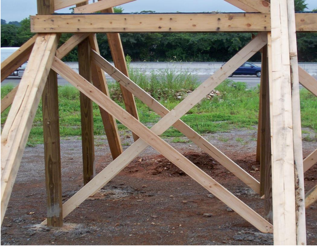
Figure 15. 2x4 X-Bracing
