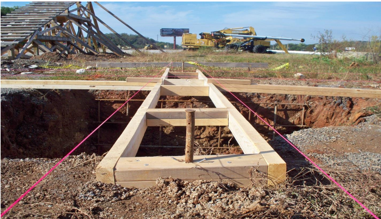
Figure 23. Nail pins securing the guide system to the ground.
