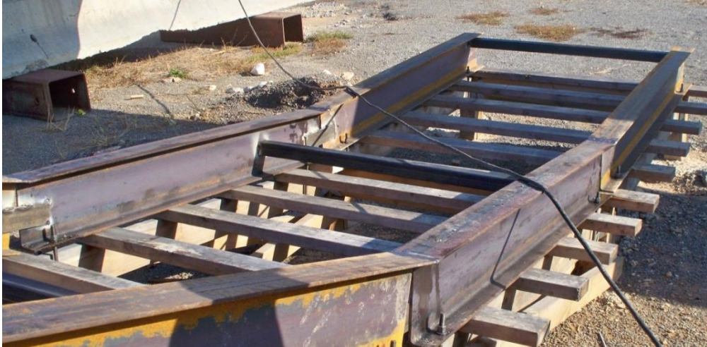
Figure 18. HSS tubes between rails.
