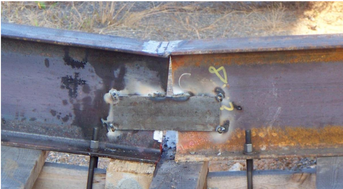
Figure 17. Welds connecting the top of the rails and splice plates.
