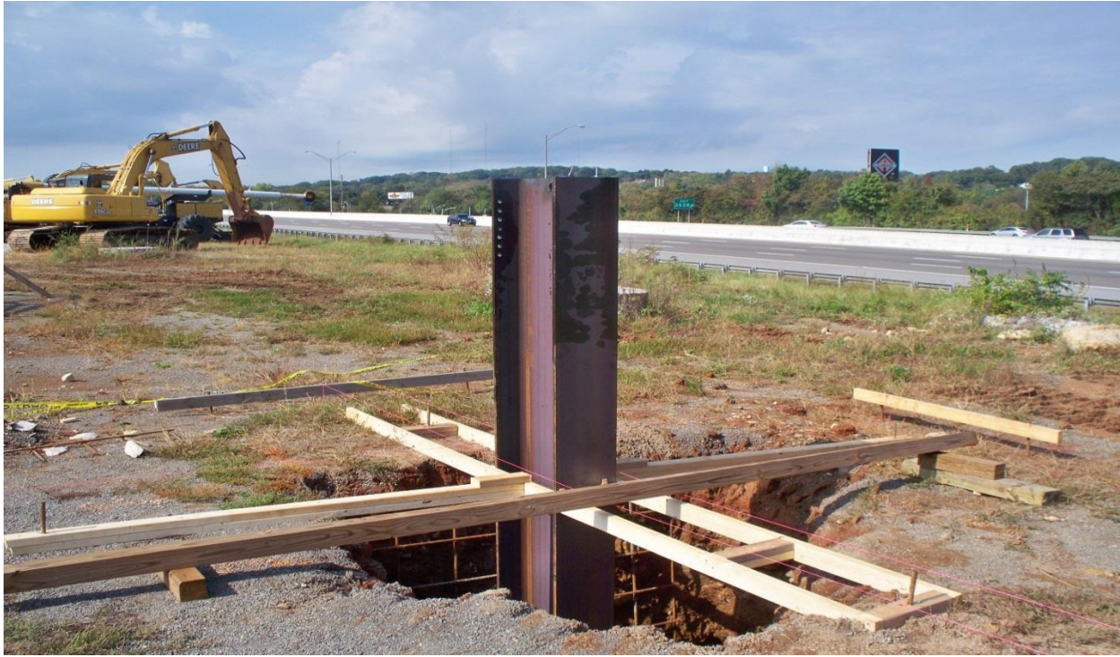
Figure 24. Steel beam sitting within the guide system.
