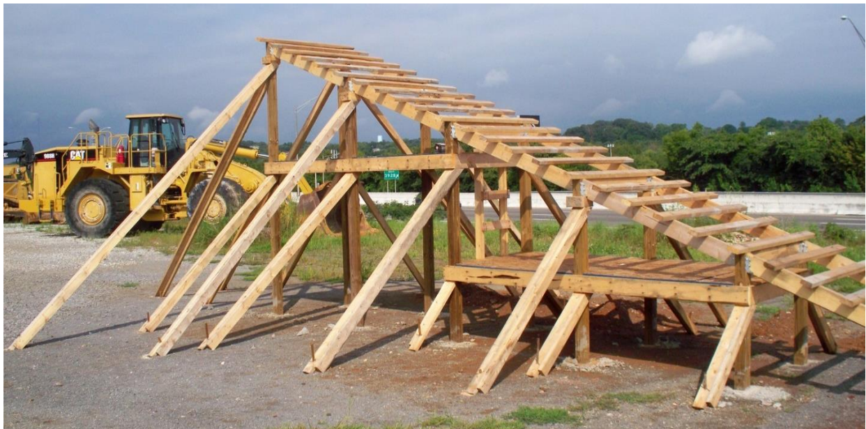
Figure 13. Lateral bracing applied at multiple levels per post.
