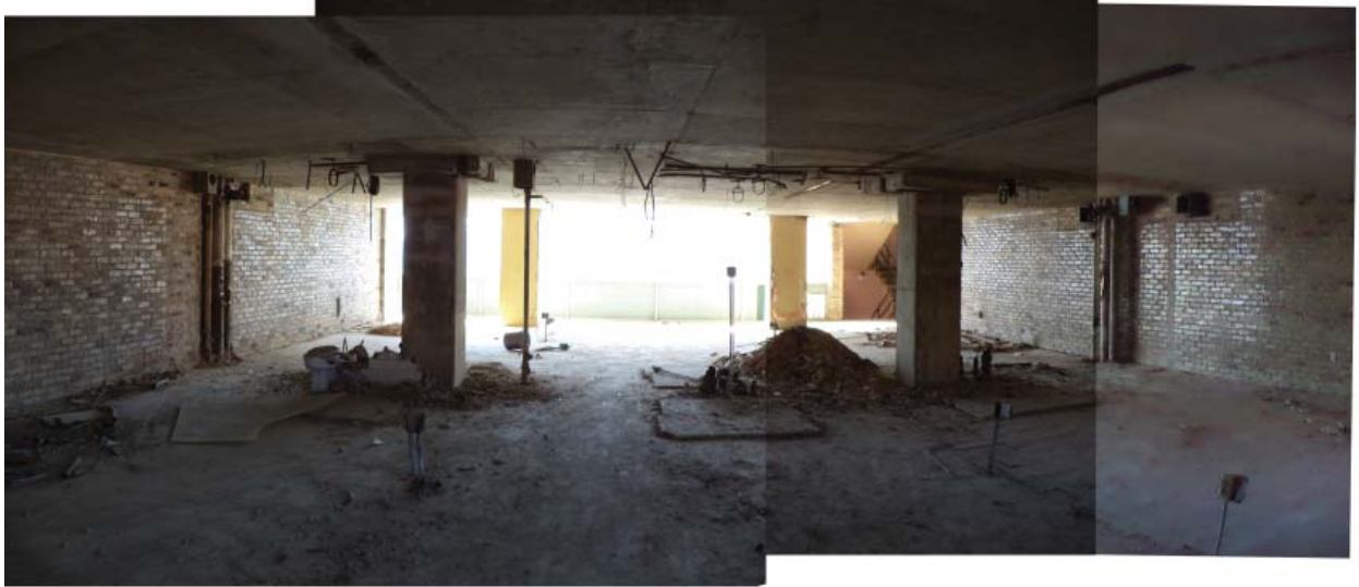
Figure 40. 1960s Annex: second floor, center. Sources: Photographs and montage by author.
