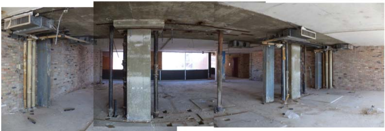
Figure 41. 1960s Annex: third floor, center. Sources: Photographs and montage by author.
