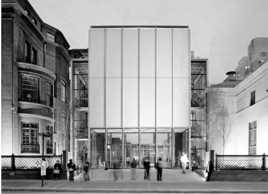
Figure 20. View of Piano's addition. Sources: Eberle, Todd and Michel Denance. Arcspace.com.
