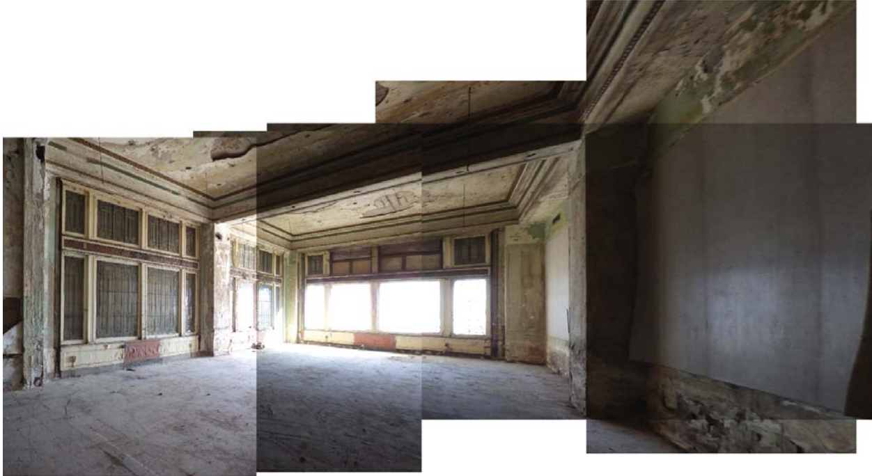
Figure 30. 1913 Hotel: Men's Lounge, ground floor. Sources: Photographs and montage by author.
