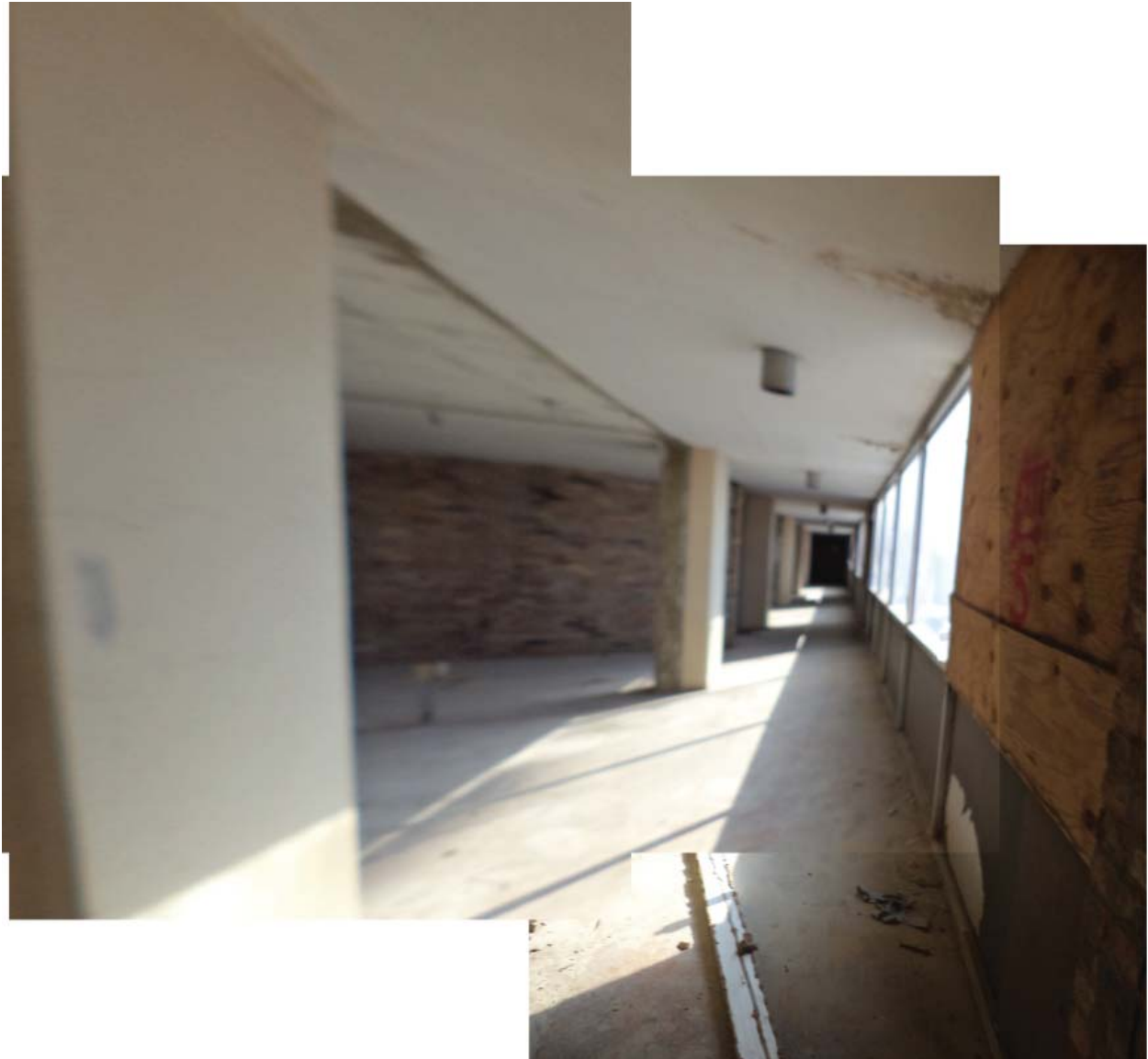
Figure 38. 1960s Annex: third floor. Sources: Photographs and montage by author.
