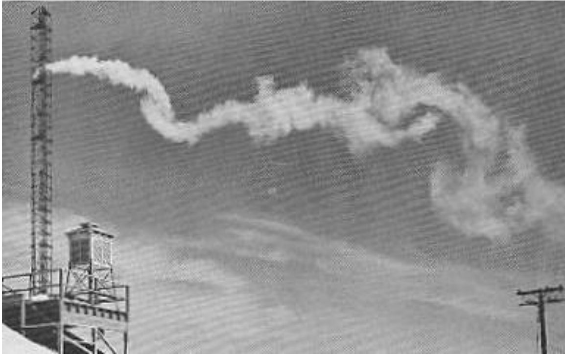
Figure 2.6 Steady state Gaussian plume from a continuous emission source
