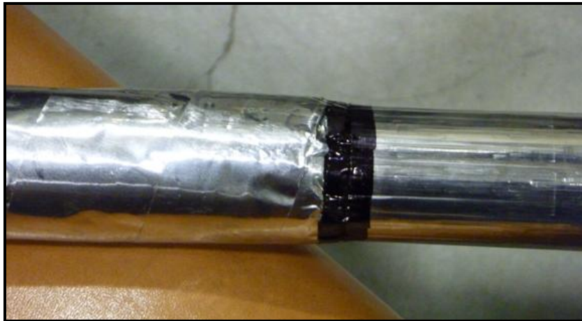
Figure 4.25: Contrasting colored band to indicate sleeve slippage
