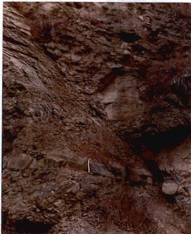
Figure 15. Closer view of one of the fractures at Field Station 55. The scale equals one foot (30.48cm).
