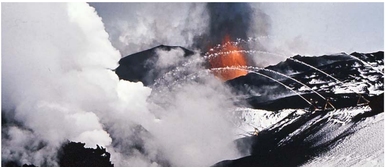
Figure 1.05 Seawater Pumping System Source: http://eldheimar.is/en/
