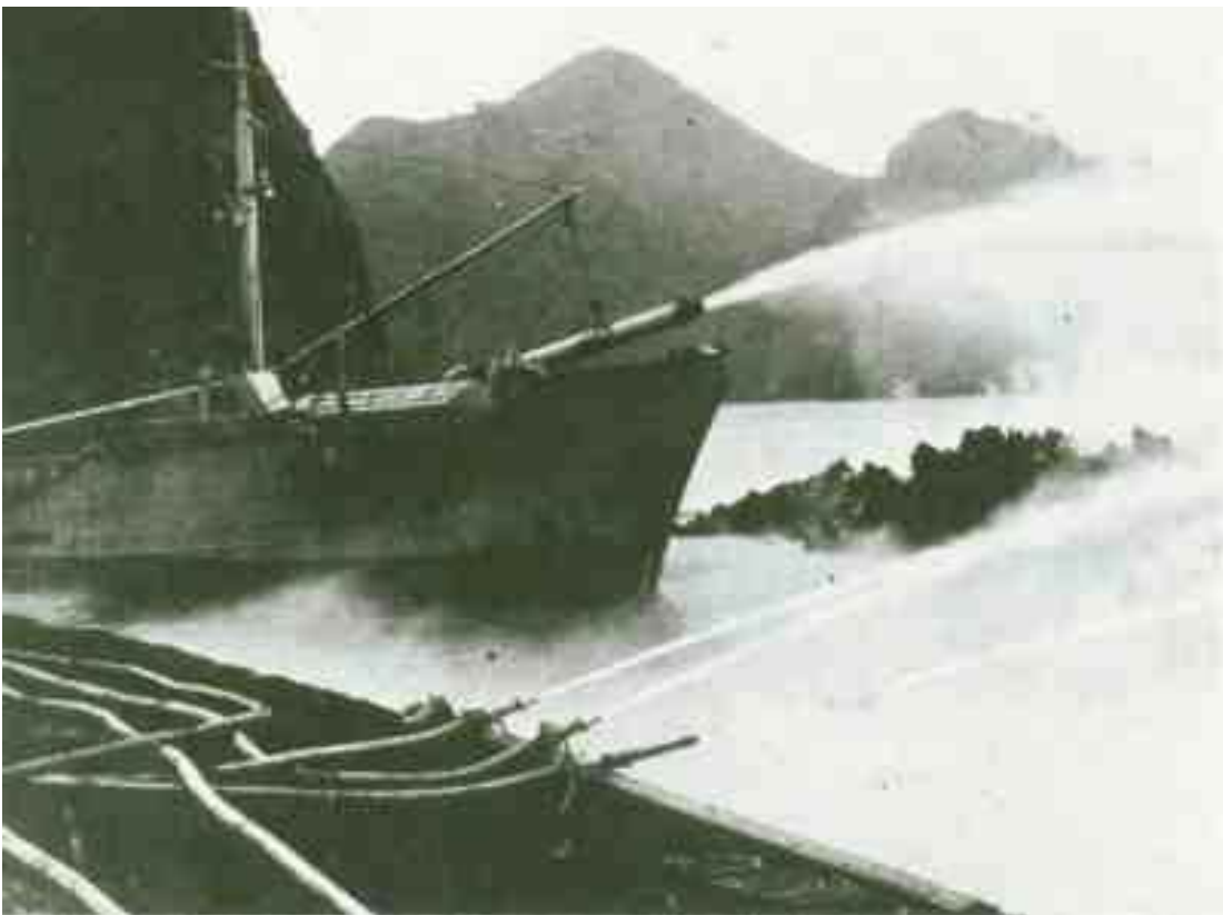
Figure 1.09 Seawater Pumping System From Boat Source: http://pubs.usgs.gov/of/1997/of97-724/32html/lavaoperations.html
