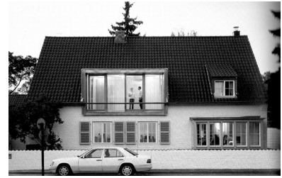
Figure 18: View of Haus Blick
