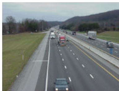
Figure 4-05. Watt Road overpass (I-40 westbound, looking east)
