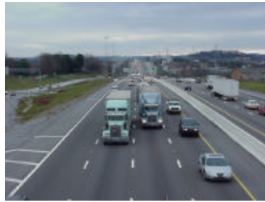
Figure 4-02. Walker Springs Road overpass (I-40 eastbound, looking west)
