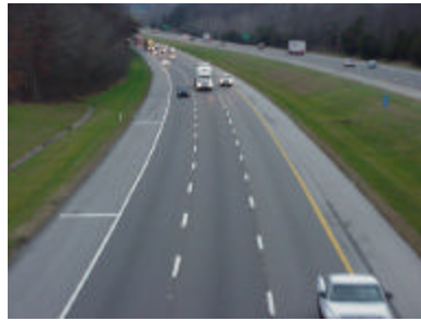
Figure 4-06. McMillan Road overpass (I-40 eastbound, looking west)
