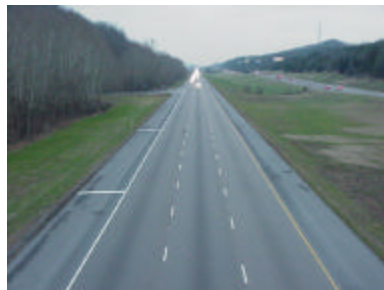
Figure 4-08. Deep Springs Road overpass (I-40 eastbound, looking west)
