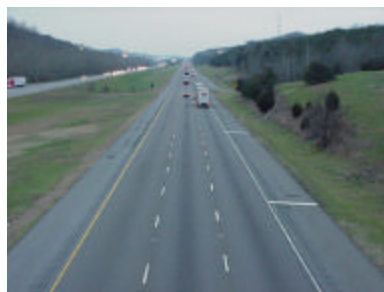
Figure 4-09. Deep Springs Road overpass (I-40 westbound, looking west)
