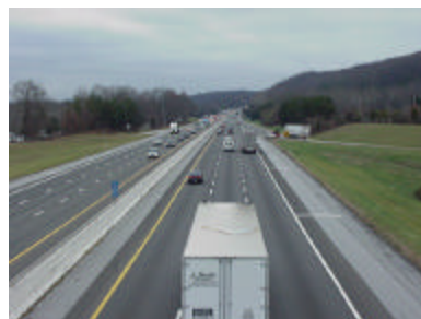
Figure 4-04. Watt Road overpass (I-40 eastbound, looking east)
