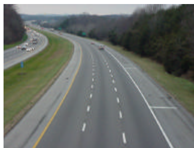
Figure 4-07. McMillan Road overpass (I-40 westbound, looking west)
