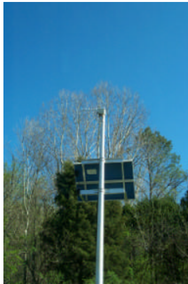
Figure 3-04. RTMS unit#1 on I-40E at milepost 369 (near Watt road overpass)
