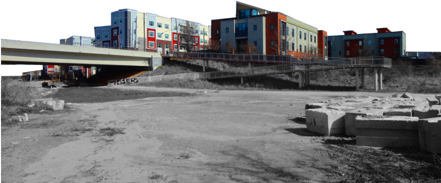
02 | Southwest Approach | Existing Condition
