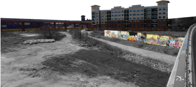
03 | Northeast Approach | Existing Condition
