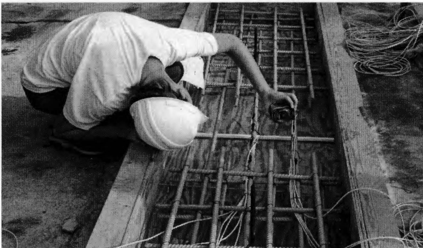
(c) Tied Rebar in Form for the Control Specimen
