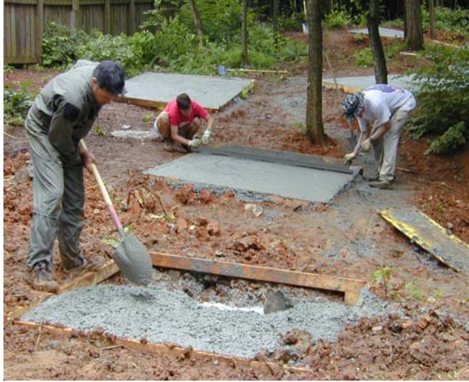
Figure 2.21~ Pouring and leveling concrete pads.
