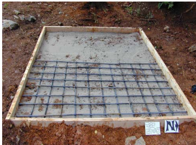
Figure 2.20~ Plot 3, leveled, with rebar distributed over eastern aspect of grave.
