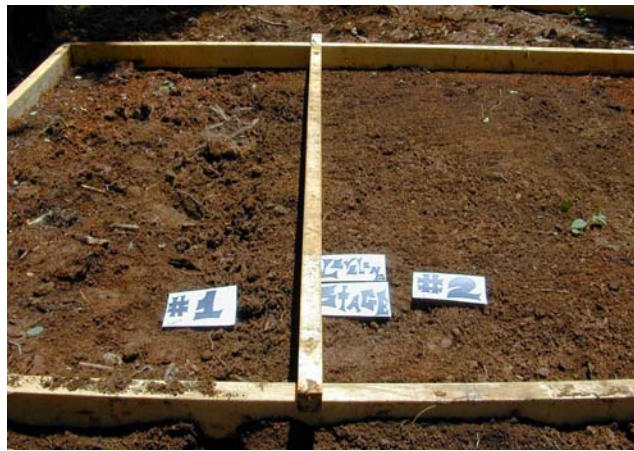
Figure 2.17~ Stages of leveling within the cement frame.
