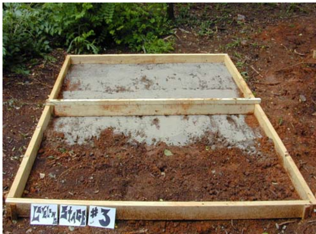
Figure 2.18~ Final leveling stage within the cement frame.
