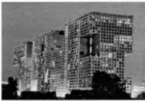
Figure 24 - Simmons Hall Exterior
