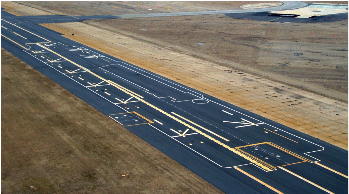
Figure 16. LHA Painted Flight Deck at NAS Patuxent River, MD
