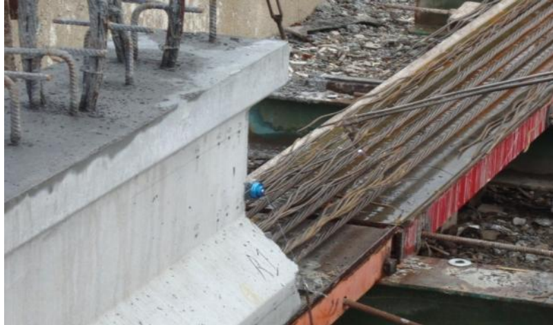
Figure 63 Release of prestress by flame cutting and unwinding of strand ends
