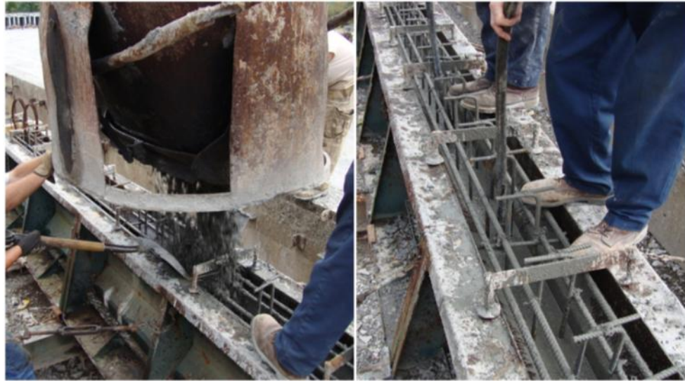
Figure 61 Placement of concrete
