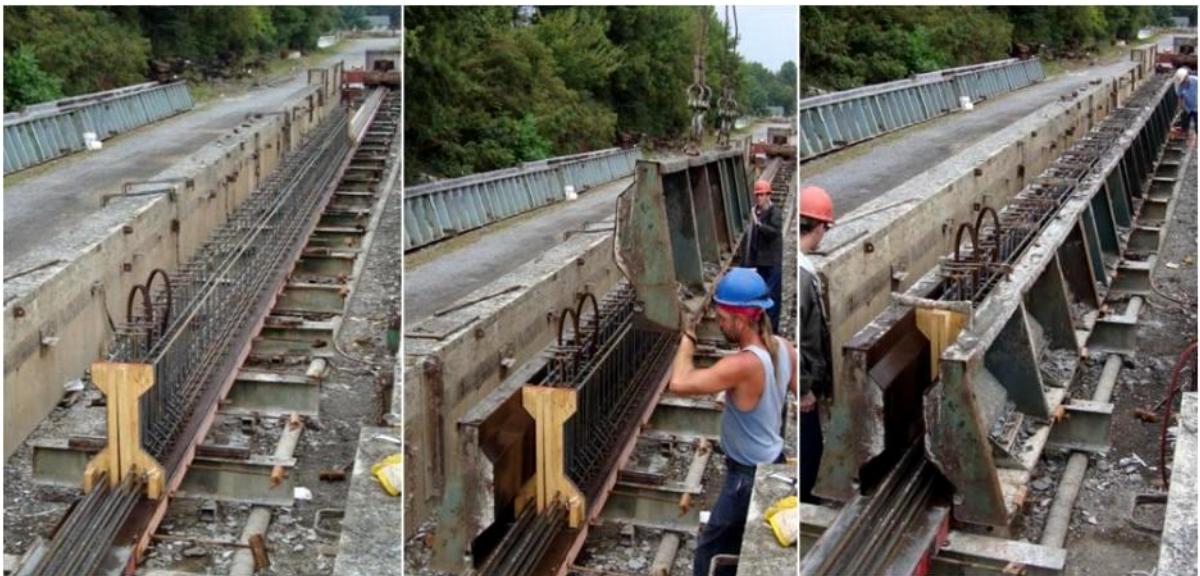
Figure 60 Placing of the side forms for the girder with 0.7 in. strand
