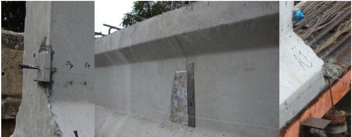
Figure 71 Deflection measurement setup at mid span
