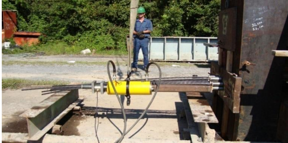
Figure 57 Strand Tensioning
