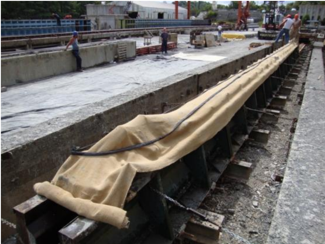
Figure 42 Water curing of girder with 0.7 inch strand
