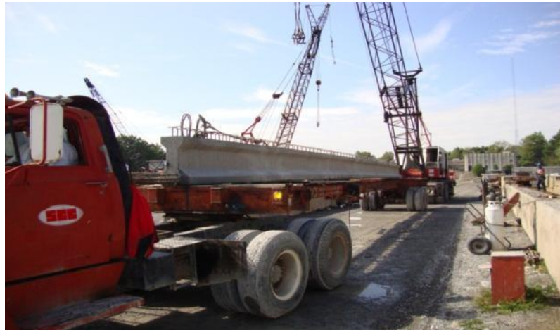
Figure 64 Moving the girder from the prestressing bed
