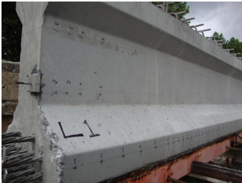
Figure 67 DEMEC points at the live end of the girder
