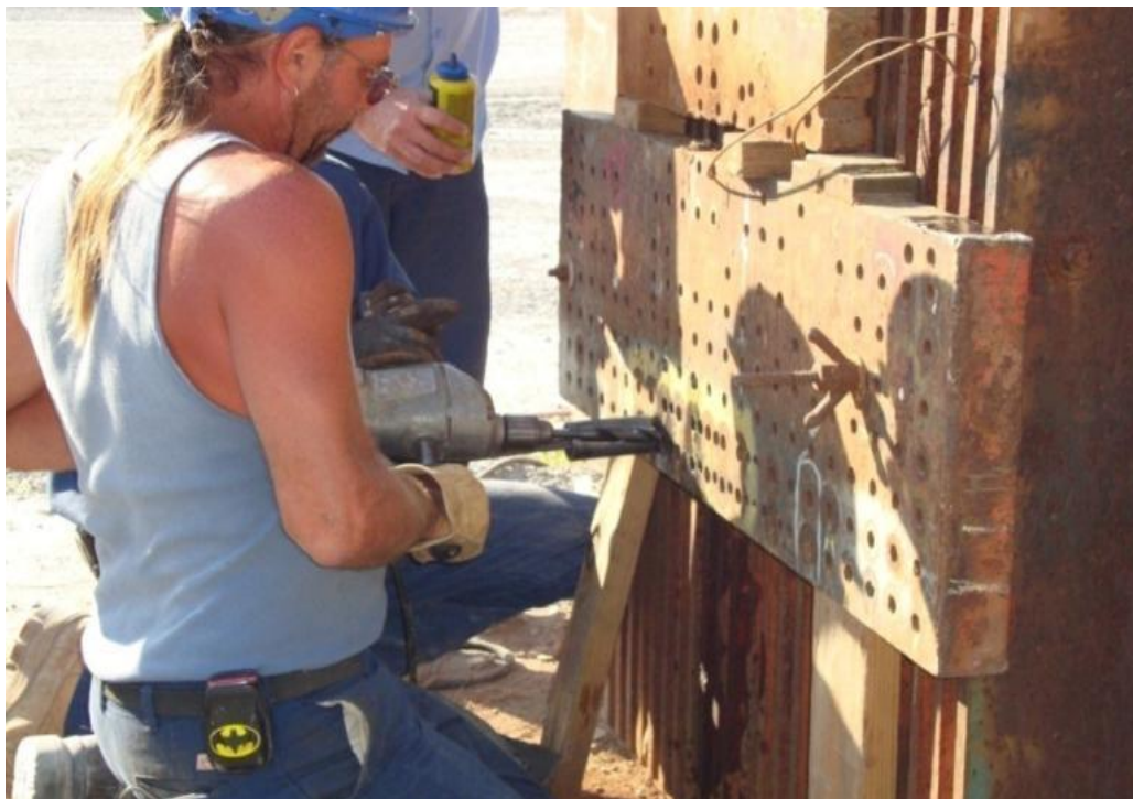
Figure 51 Increasing the diameter of the holes in the bed
