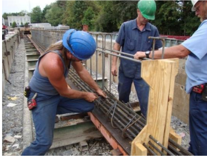
Figure 59 Tying of mild steel reinforcement for the girder
