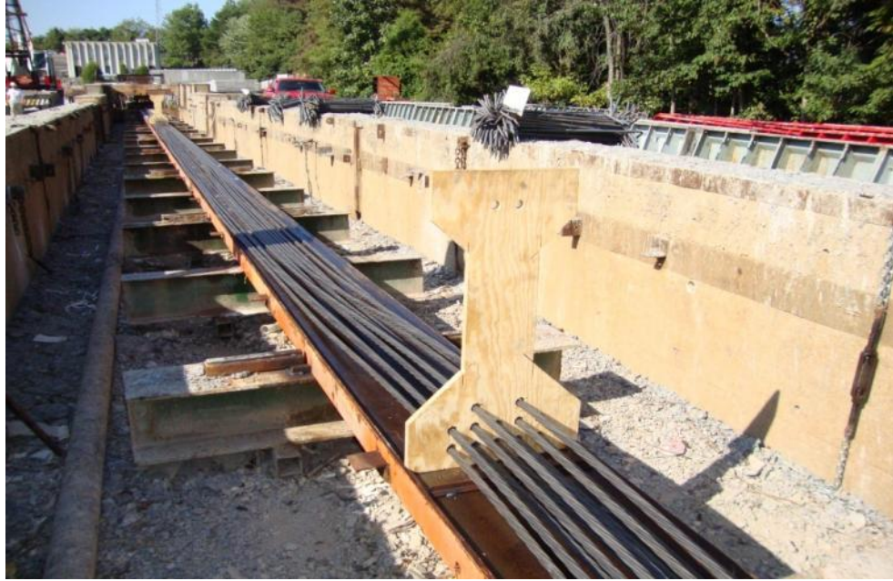
Figure 54 12 Nos. of 0.7 in. strands before tensioning
