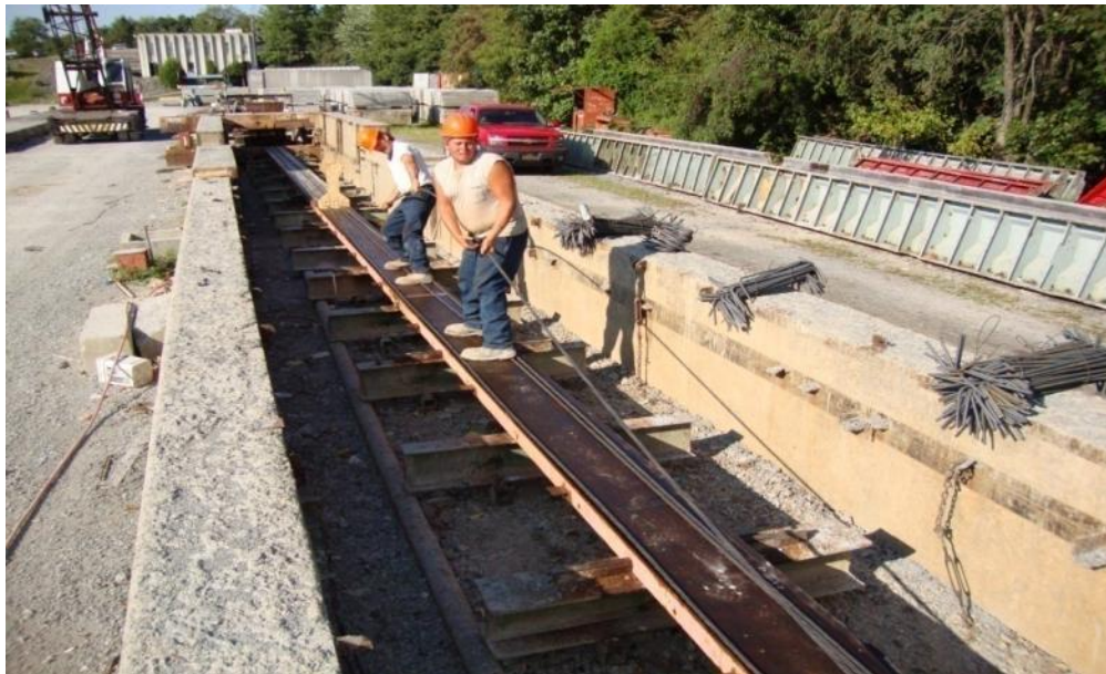
Figure 53 Ross prestress personals laying down the 0.7" strands
